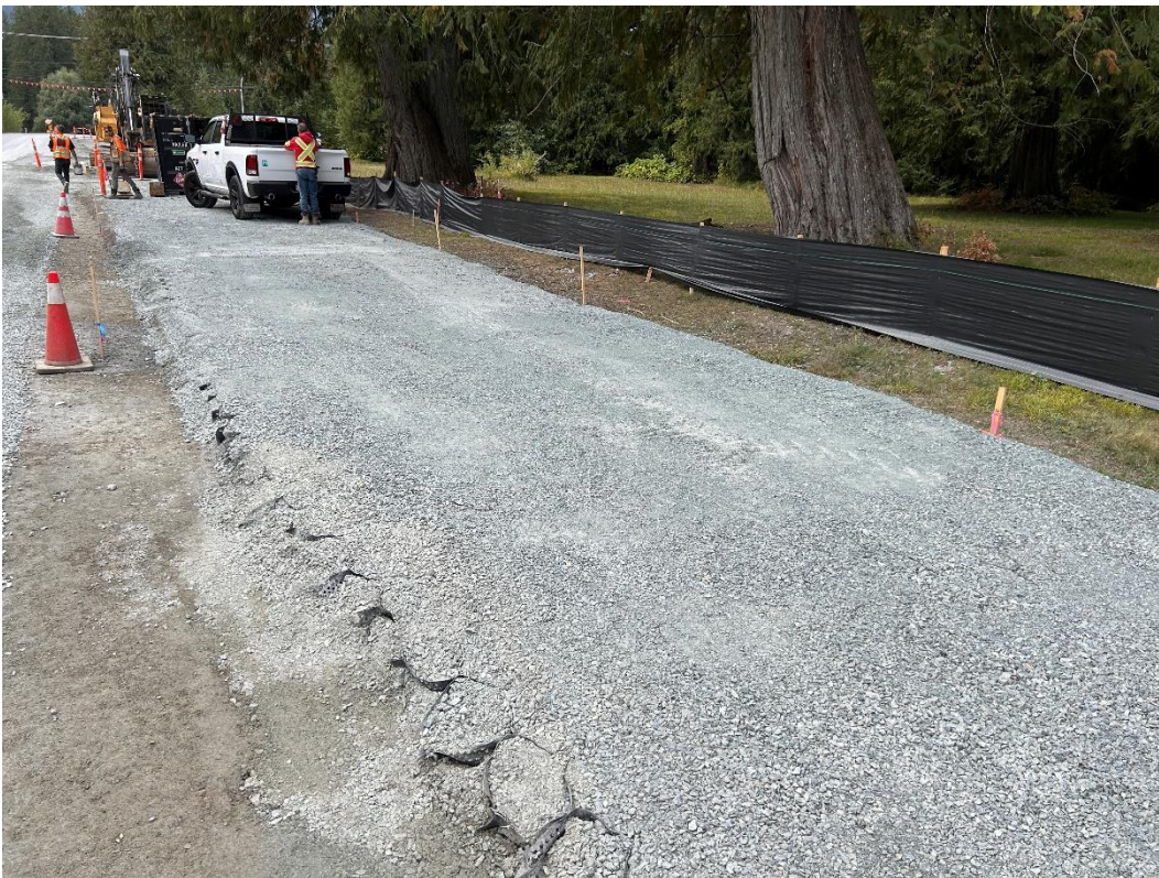
Figure 4 – Geocell textile used to reduce compaction on root systems for Friendship trail construction
