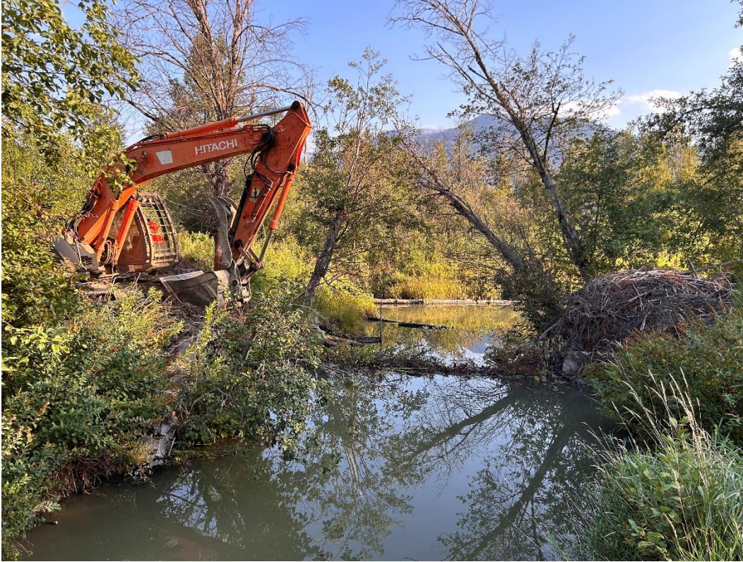
Figure 3 – One Mile Lake outlet channel beaver dam removal
