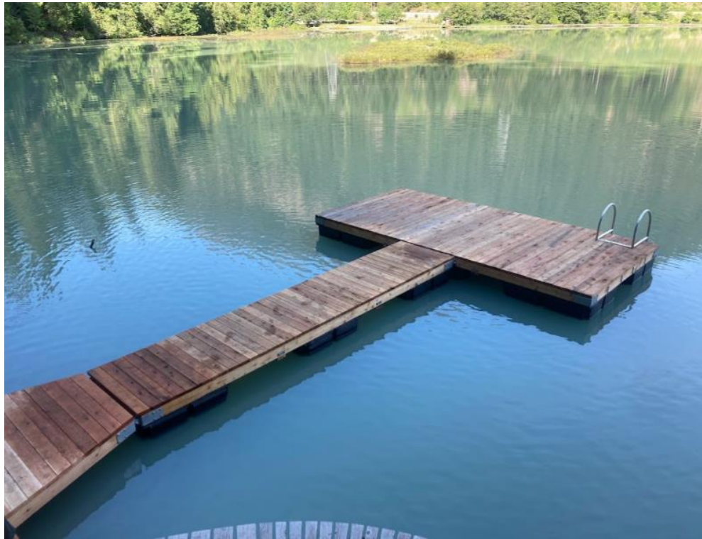
Figure 7 – One Mile Lake floating dock replacement
