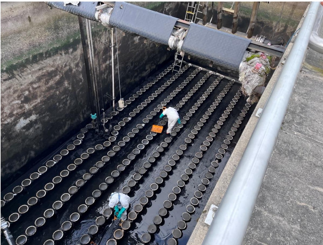
Figure 6 – WWTP Basin cleaning
