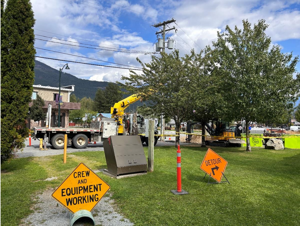
Figure 5 – Construction commencing on Aster St Level 3 EV charging stations
