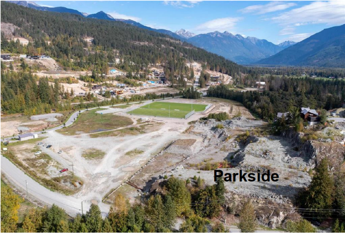
Looking East at Site
