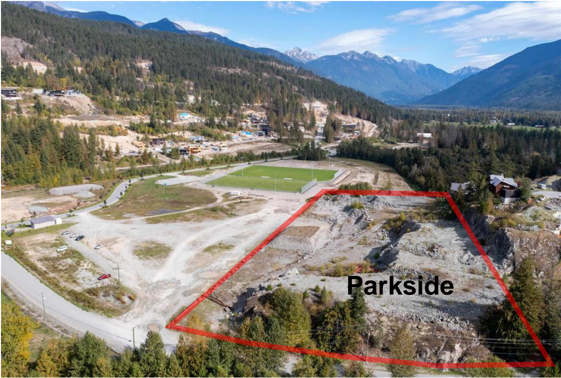
Looking East at Site
