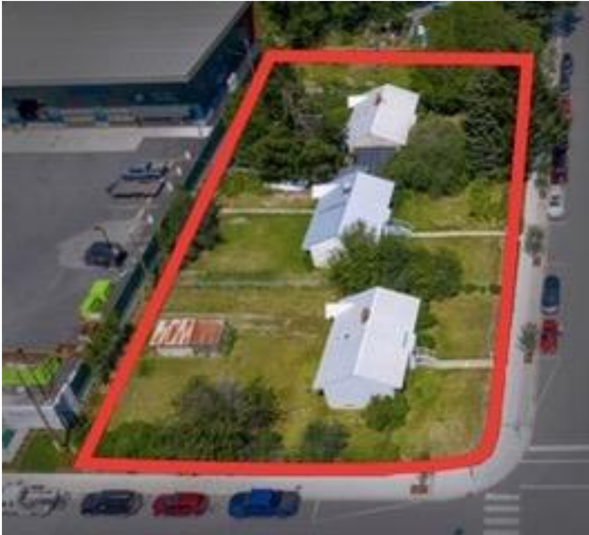
aerial view showing existing three buildings across property
