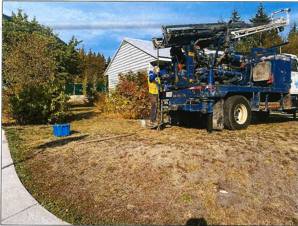
Photograph 1 – Drilling BH-02 on October 7, 2022 looking north-west
