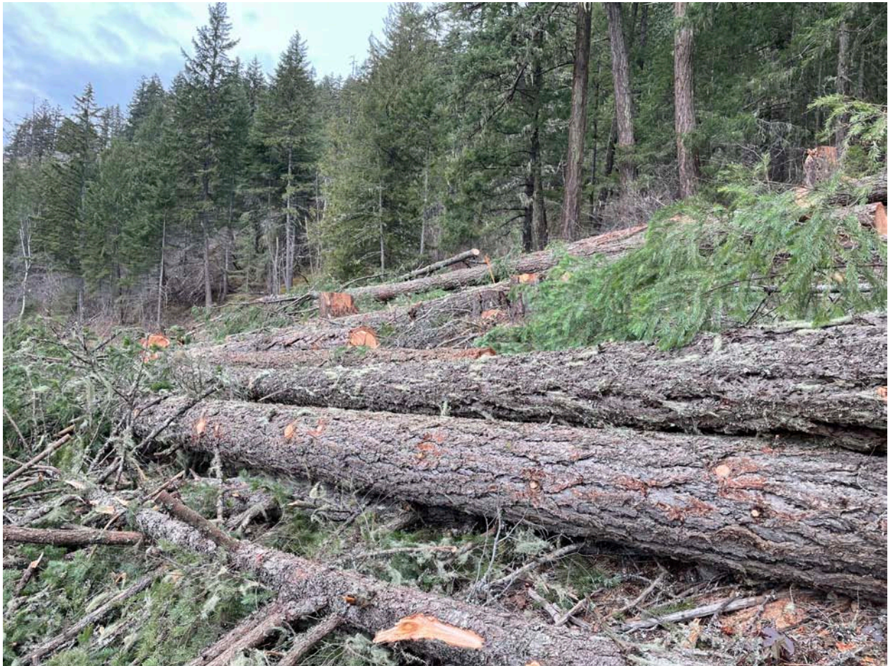
Fell and Buck Douglas fir during Road G clearing
