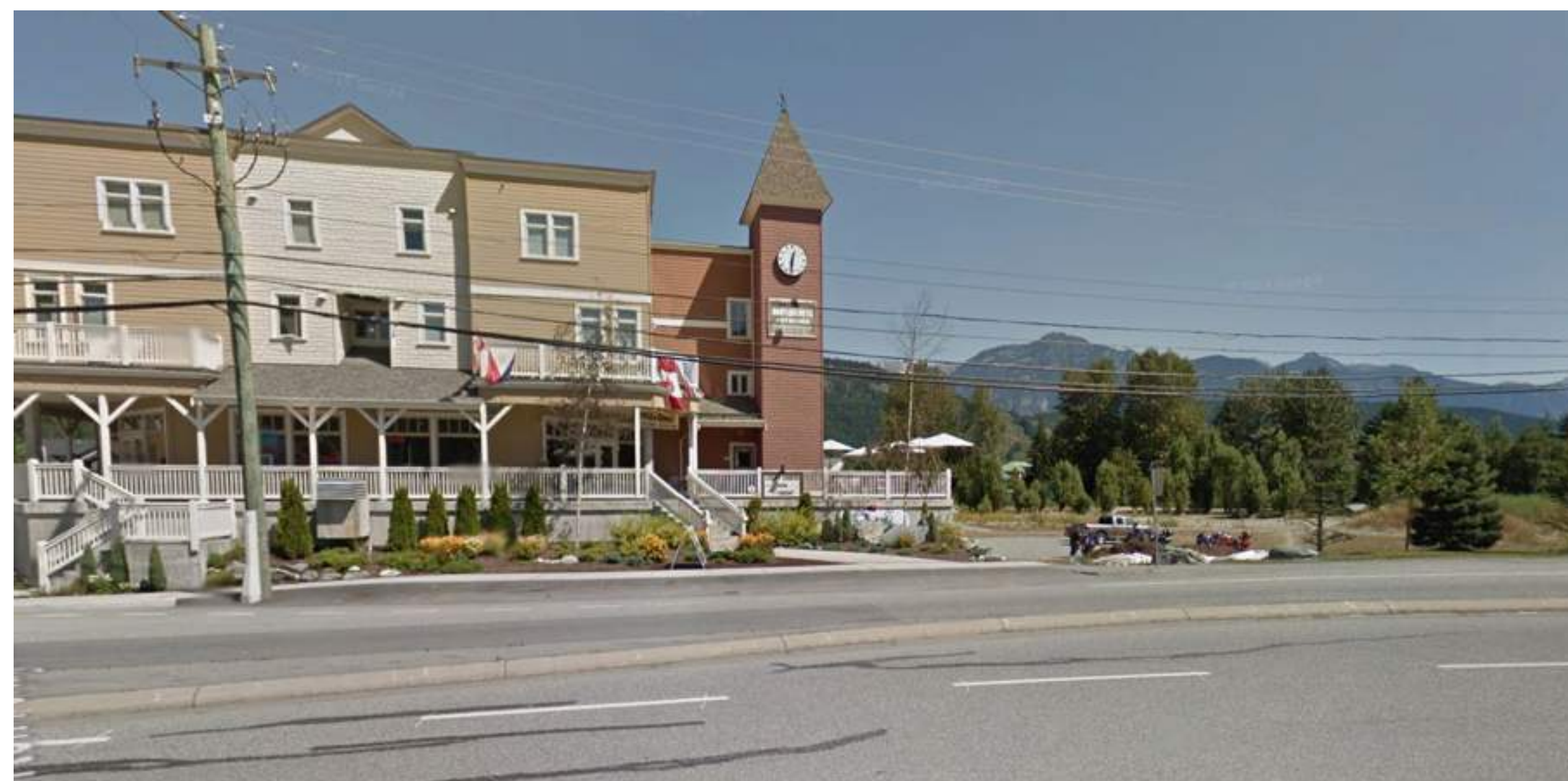
3 VIEW FROM PEMBERTON PORTAGE RD FACING EAST
