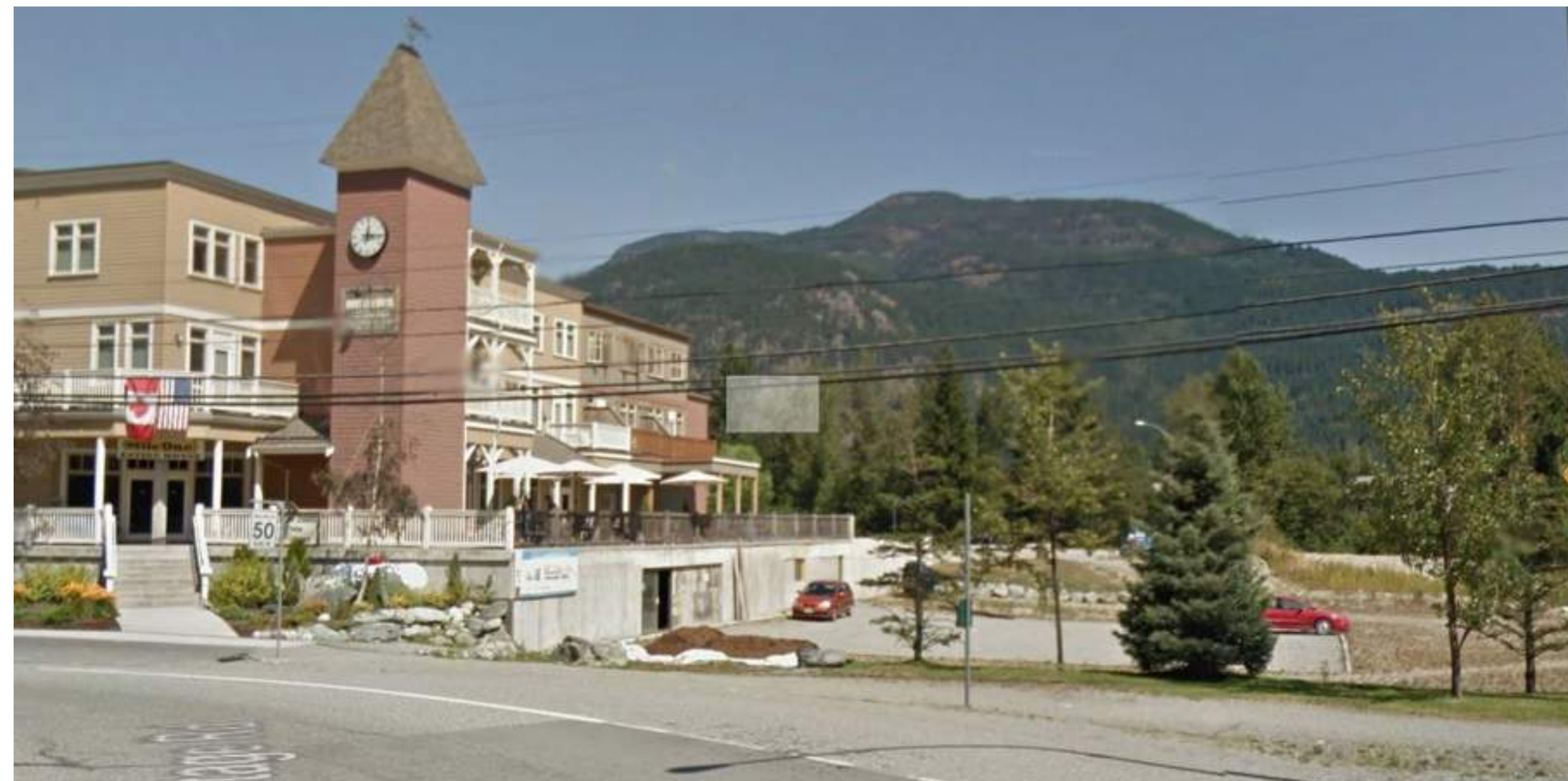
1 VIEW FROM PEMBERTON PORTAGE RD FACING NORTH
