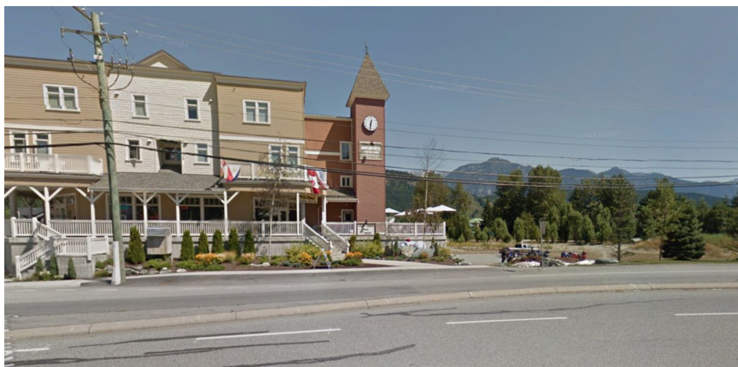
3 VIEW FROM PEMBERTON PORTAGE RD FACING EAST
