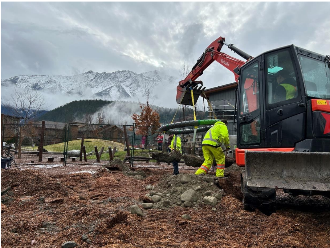
Figure 1 – Nature Play playground removal for site preparations of Daycare Expansion
