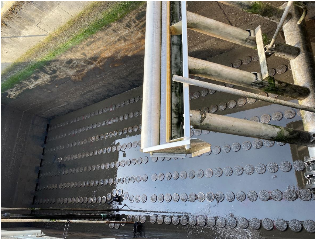
Figure 3 – WWTP Basin Cleaning
