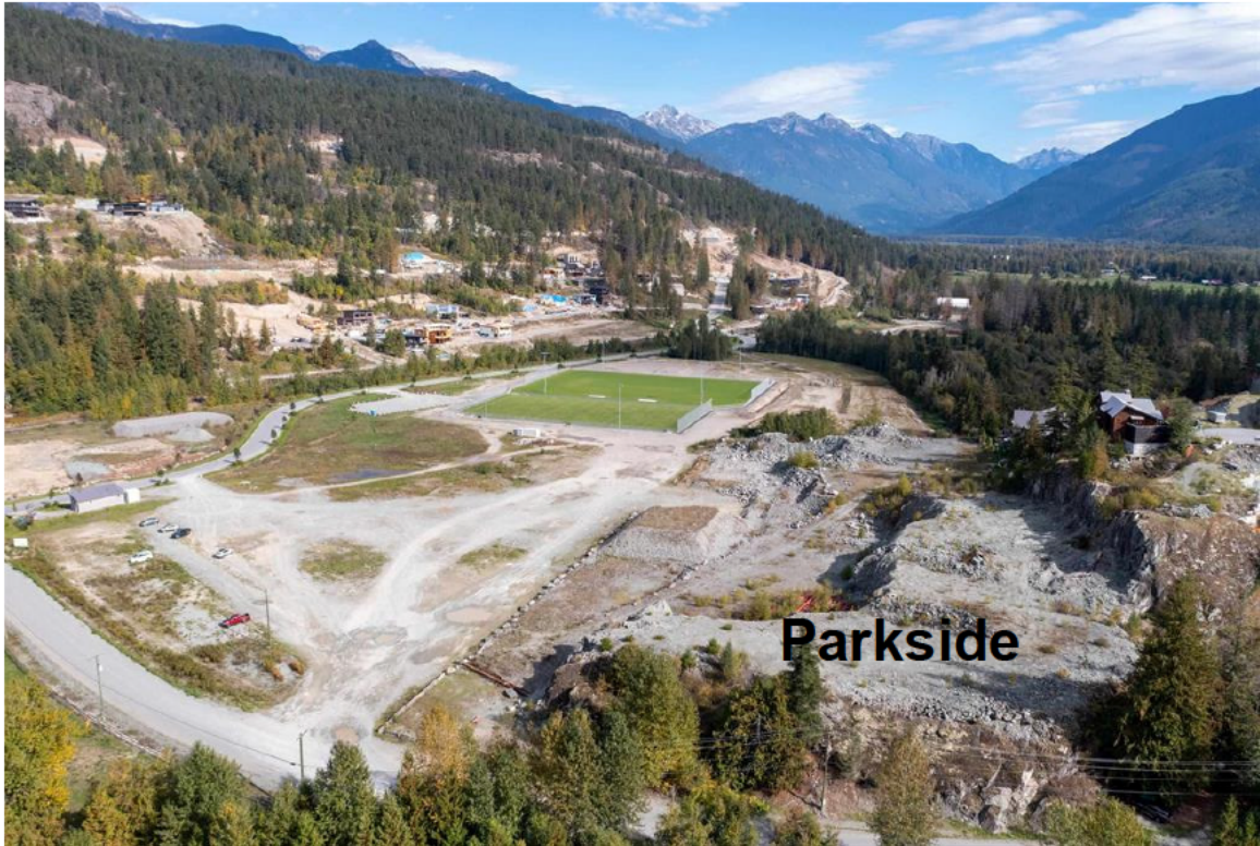
Looking East at Site
