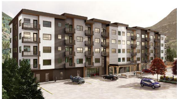
VIEW OF FRONT ENTRANCE
