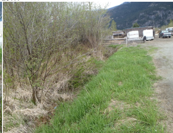
Photo 12: View of the ditch along Prospect Street. April 26, 2017.
