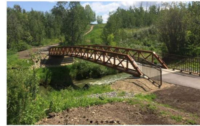
EXAMPLE OF STEEL TRUSS BRIDGE (REFERENCE IMAGE: BEAR CREEK BRIDGE IN GRANDE PRAIRIE, ALBERTA)
