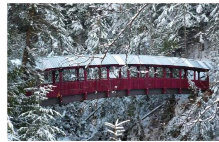
EXAMPLE OF COVERED STEEL PLATE GIRDER BRIDGE (REFERENCE IMAGE: KASLO TRAIL PEDESTRIAN BRIDGE IN KASLO, BC)
