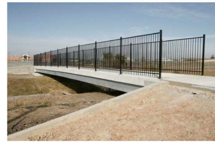
CONCRETE BOX BEAM/SLAB BRIDGE
