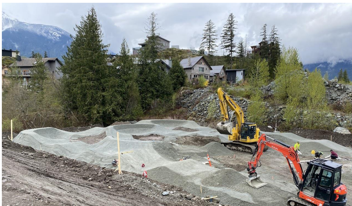
Figure 1 – Bike Skills Park Pump track construction
