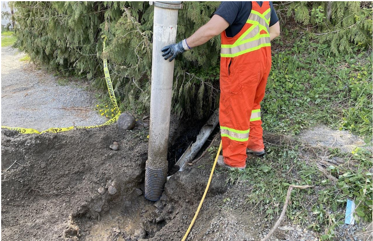
Figure 5 – Sewer service line emergency repair – beside general store
