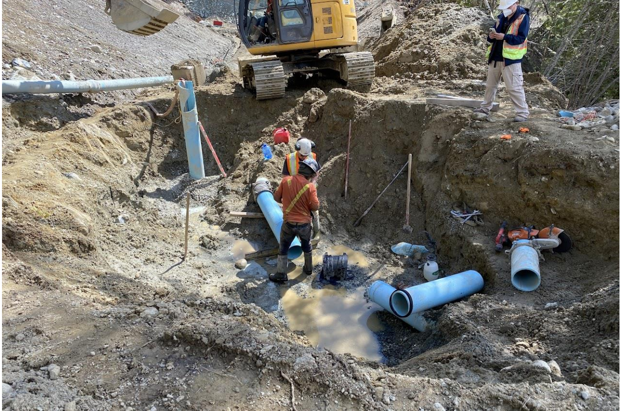
Figure 4 – Water main connection for Sunstone Phase 2
