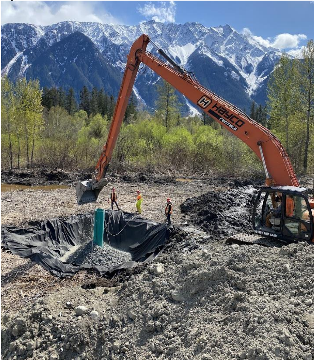
Figure 2 – Storm Pond Irrigation wet well construction at Den Duyf Park
