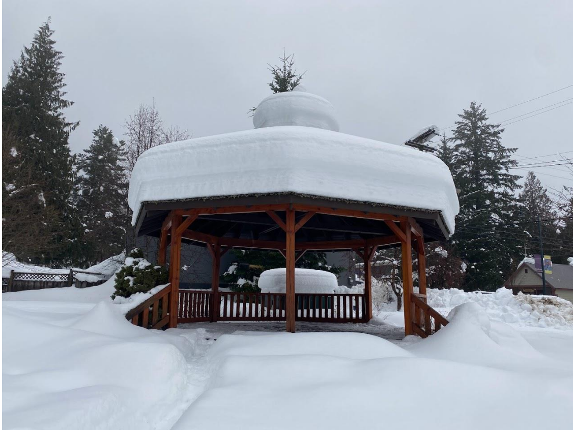
Figure 2 – Snow load on gazebo roof at Pioneer Park
