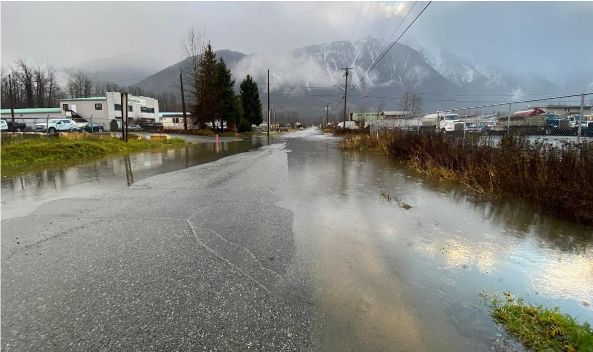
Figure 3 – Flooding in the Industrial Park
