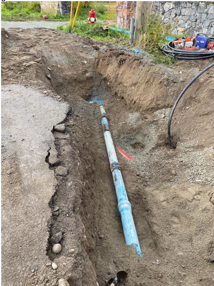
Figure 1 – Old Mill Rd Water main / service line repair
