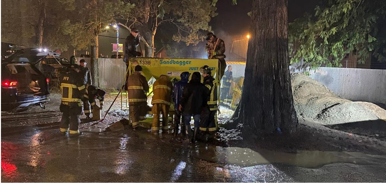
Figure 4 – Sandbag station during flooding events
