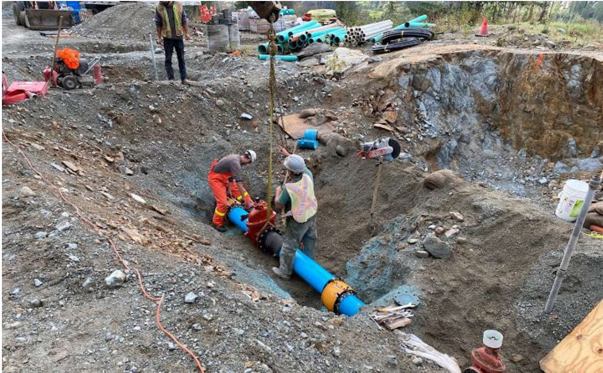
Figure 6 – Sunstone Phase 1C water main tie-in (Cerulean Dr)
