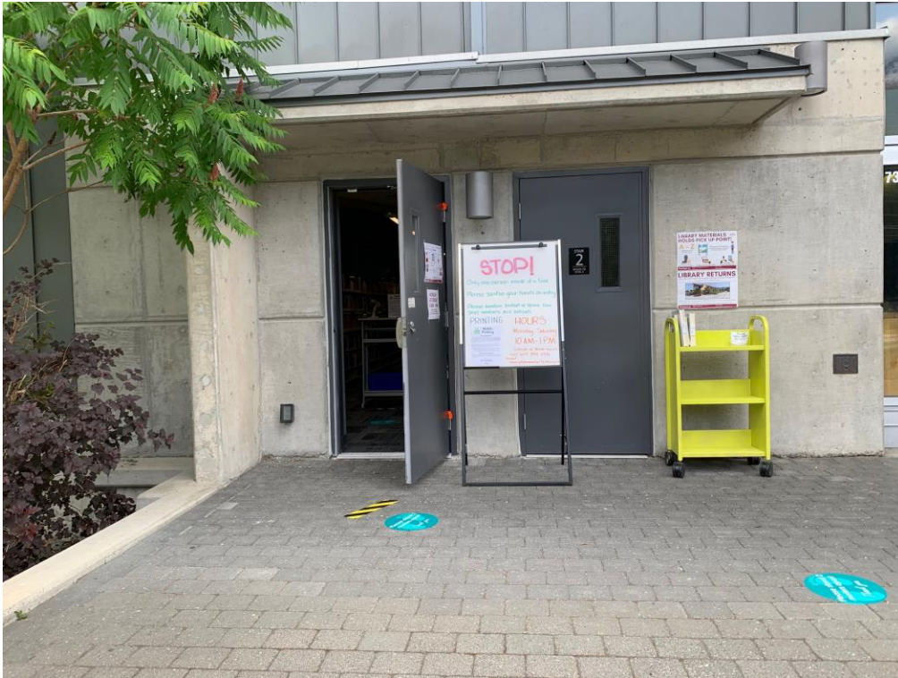
Existing Library Fire Exit – South side of Building
