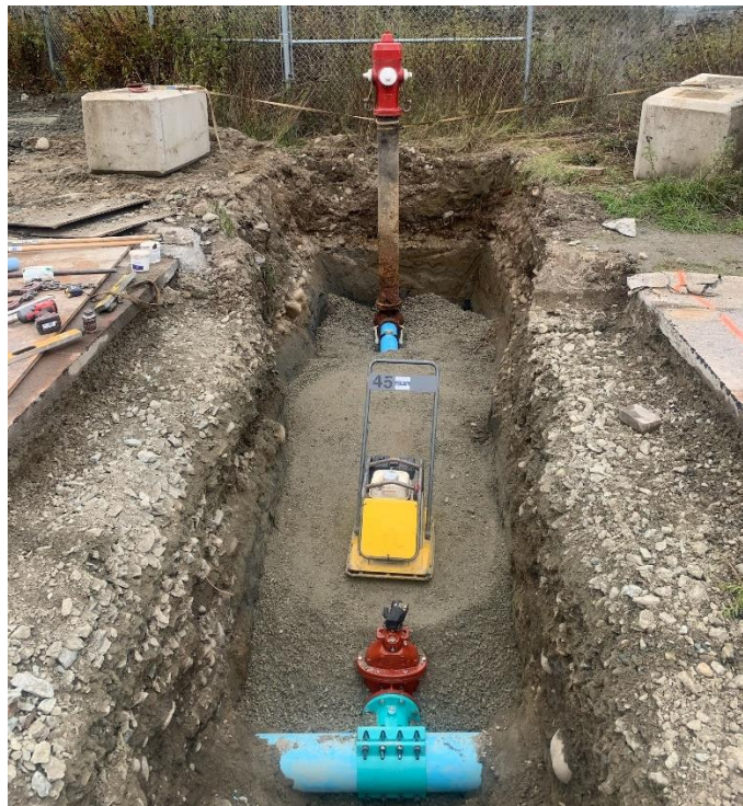
Figure 7 – Fire Hydrant relocation – Carpenter Rd (Industrial Park)
