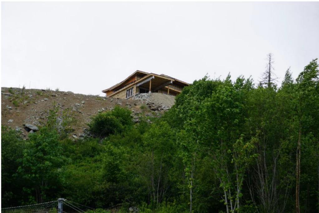
Figure 10 – Local retaining wall example 4 of 6. Example of 1H:1V slope. Although considered acceptable, this solution is not aesthetically pleasing, and prone to erosion. Terraced retaining provides better vegetation cover, less erosion, and a more pleasing appearance. Viewed from Sunstone Development.
