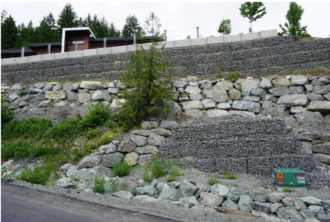
Figure 8 – Local retaining wall example 2 of 6. Walls over height but including terrace for planting. Location: main access to The Ridge.
