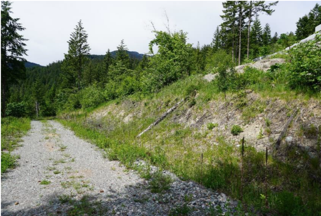
Figure 3 – Current conditions at southern property line looking west.
