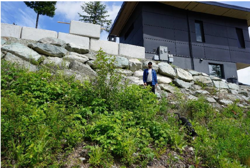
Figure 6 – Center lot facing west showing relative scale of the neighbouring property's retaining. Example of existing wall more than 1.2m in height.
