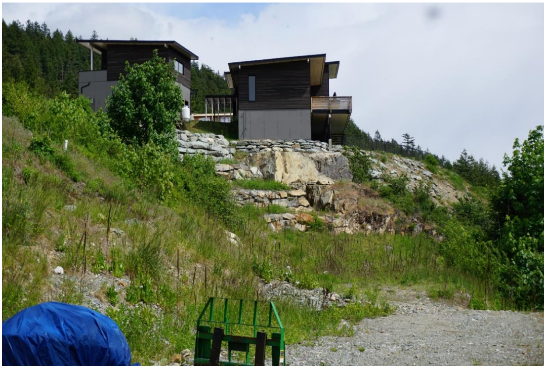
Figure 6 – Local retaining wall example 1 of 6. Example of well executed terraced walls. Location: The Ridge.
