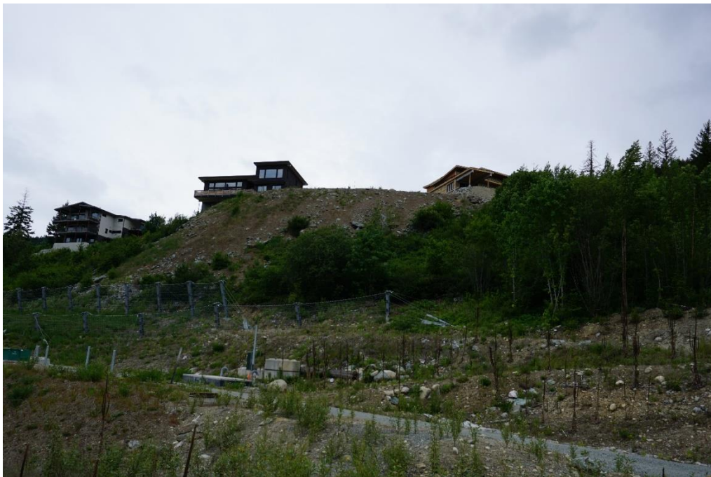
Figure 10 – Local retaining wall example 5 of 6. Example of an unretained slope. Viewed from Sunstone Development.
