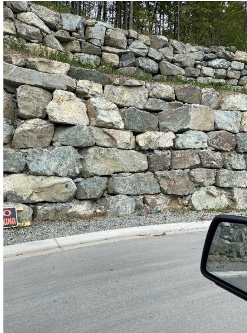
Figure 11 – Local retaining wall example 6 of 6. Developer built wall in Sunstone for road access. As all hillside developments will require road access, so do homes. Lots sloping in two directions require retaining across the slopes from a high wall to a low wall in order to use the lot efficiently.
