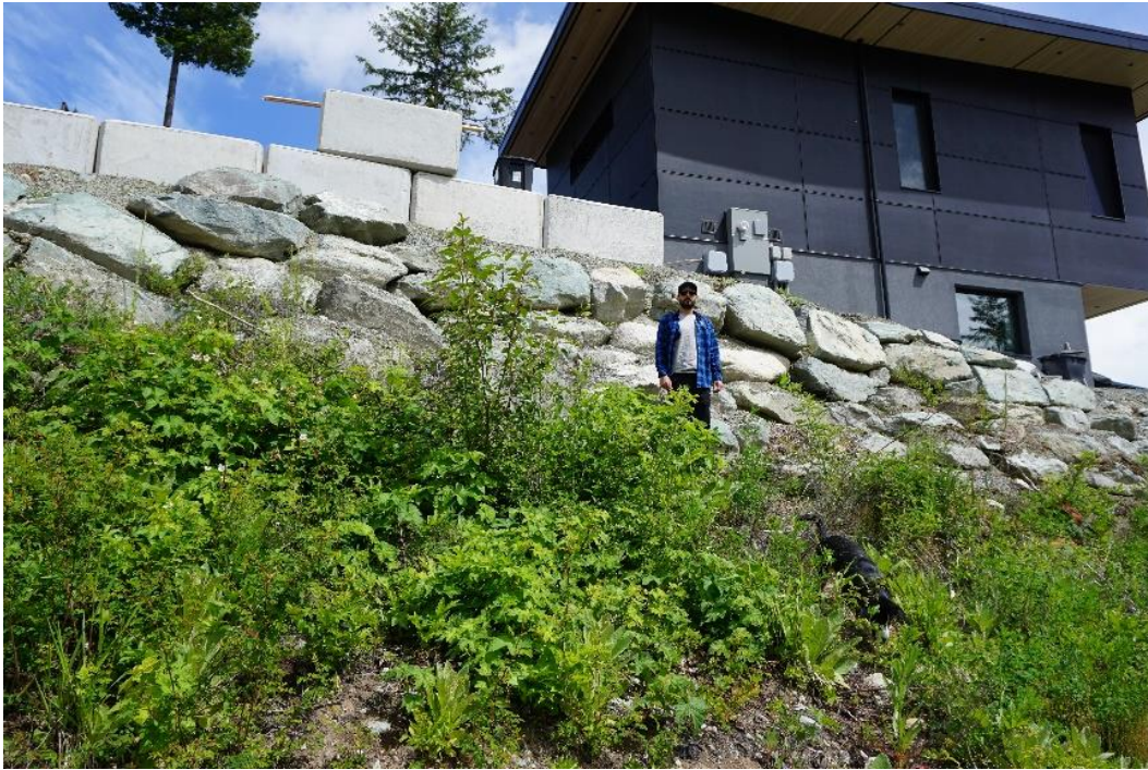
Figure 5 – Neighbouring Lot 7, facing west showing relative scale of a neighbouring property's retaining. Example of existing wall more than 1.2m in height.
