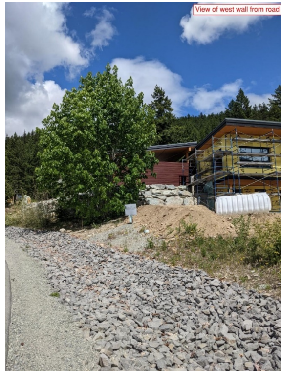
Figure 2: View of West Wall from Road
