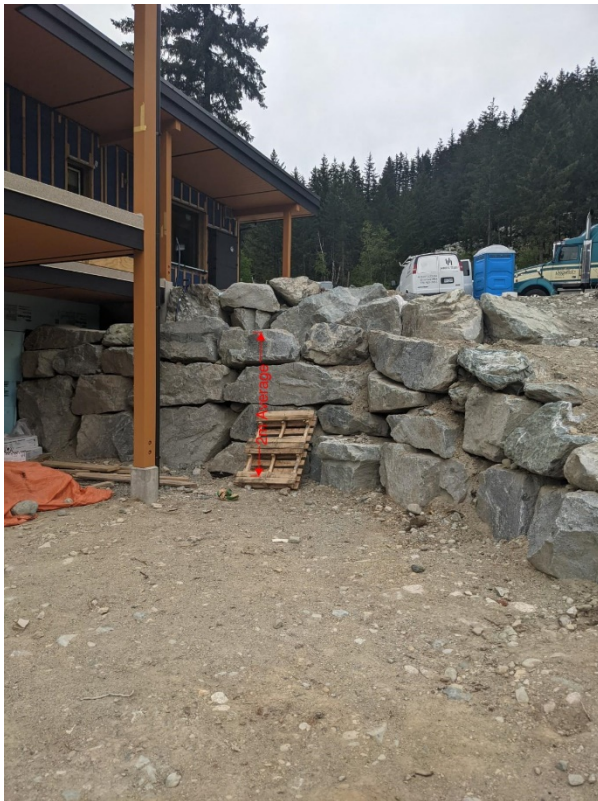
Figure 1: View of East Wall
