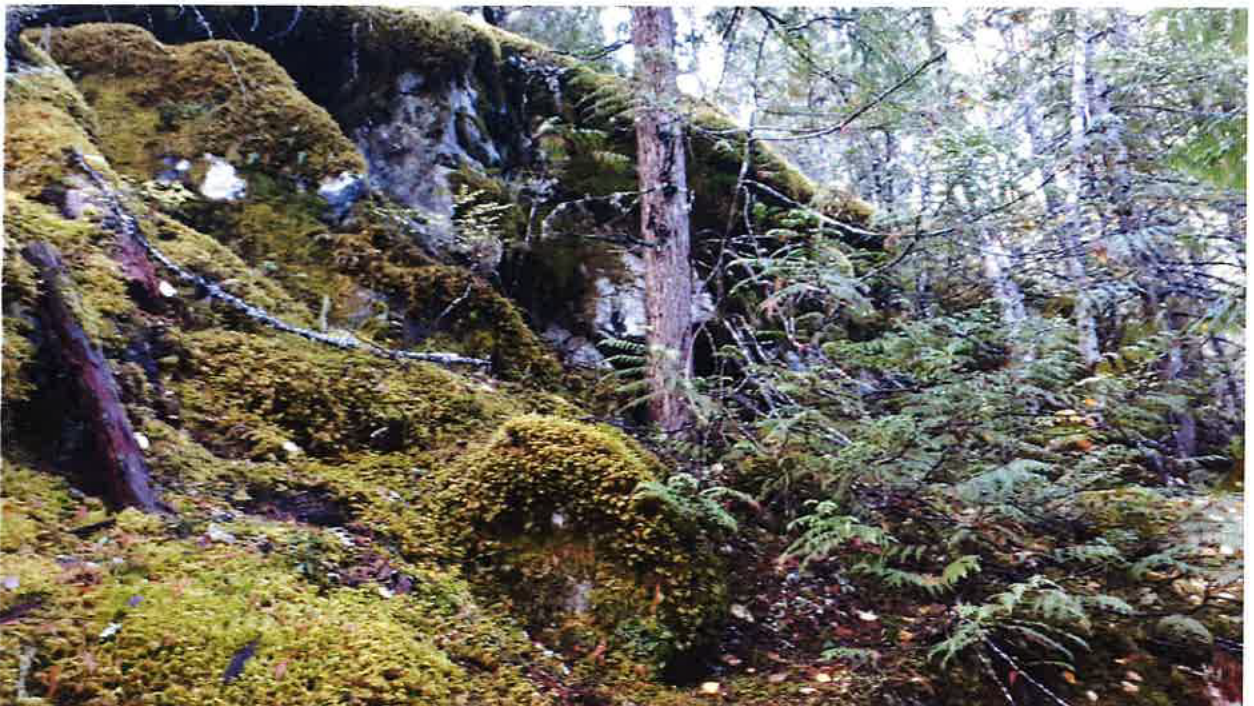
Photograph 12 – Bedrock Bluff Rockfall Source – P11
