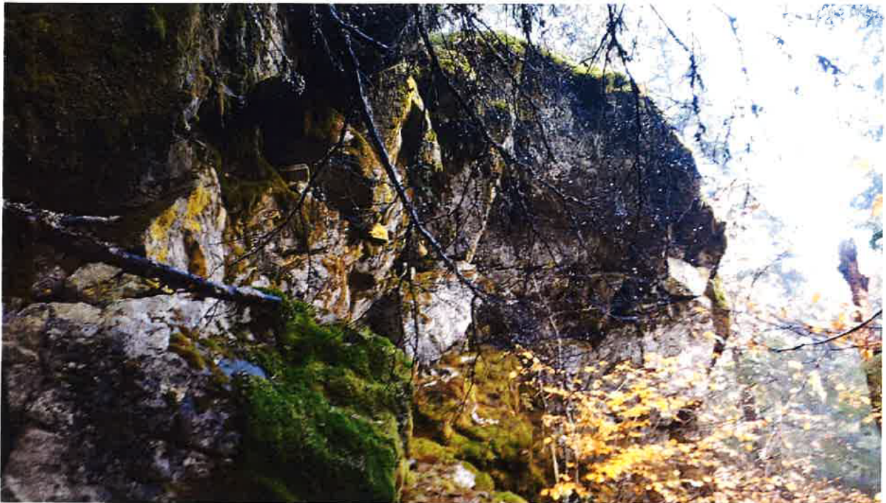
Photograph 3 – Overhanging Bluff, Rockfall Source– P3
