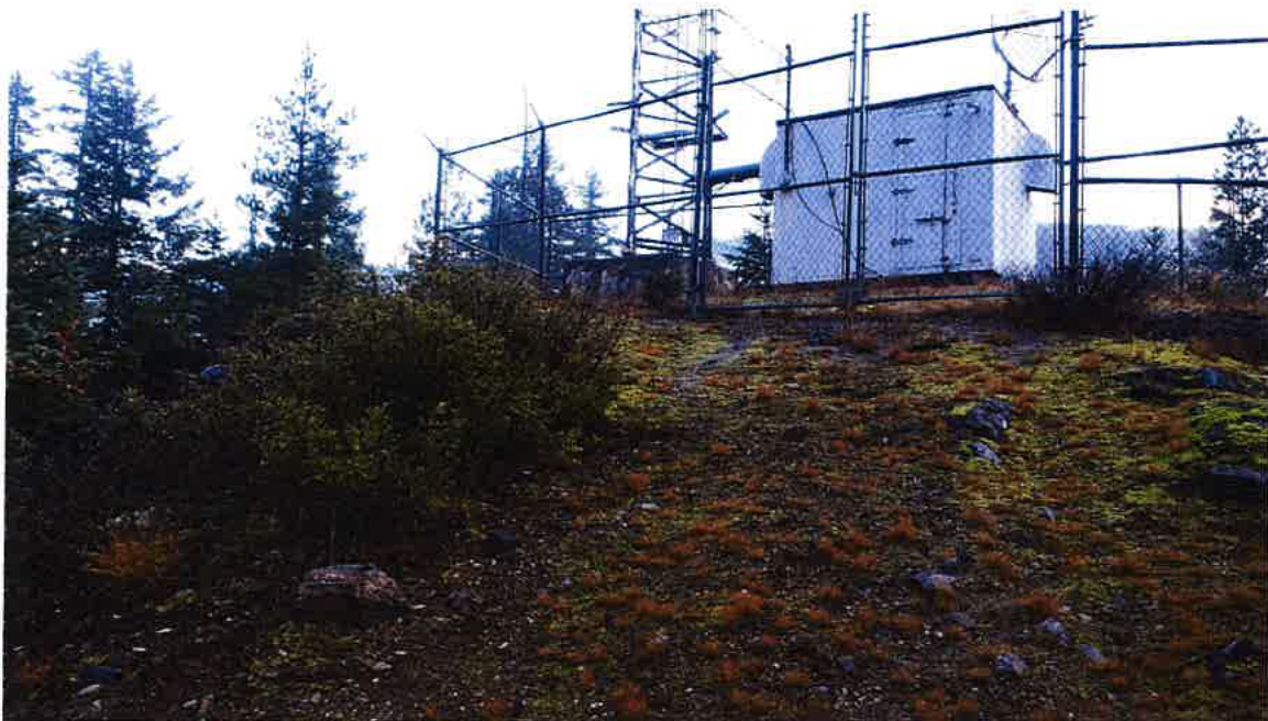
Photograph 2 – Communication Towers – P2
