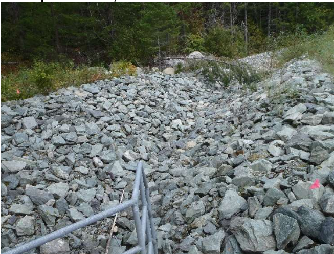
Photo 11: View of the armored section of Watercourse #3. September 10, 2019.
