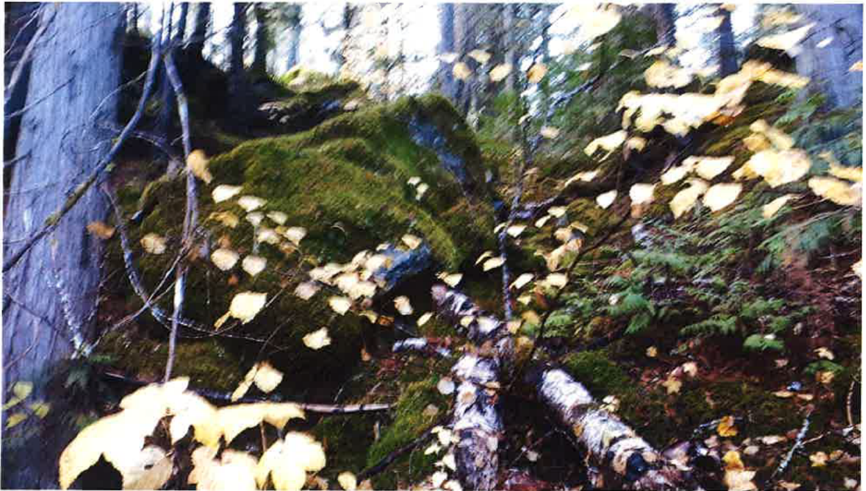
Photograph 9 – Loose Boulders – P8
