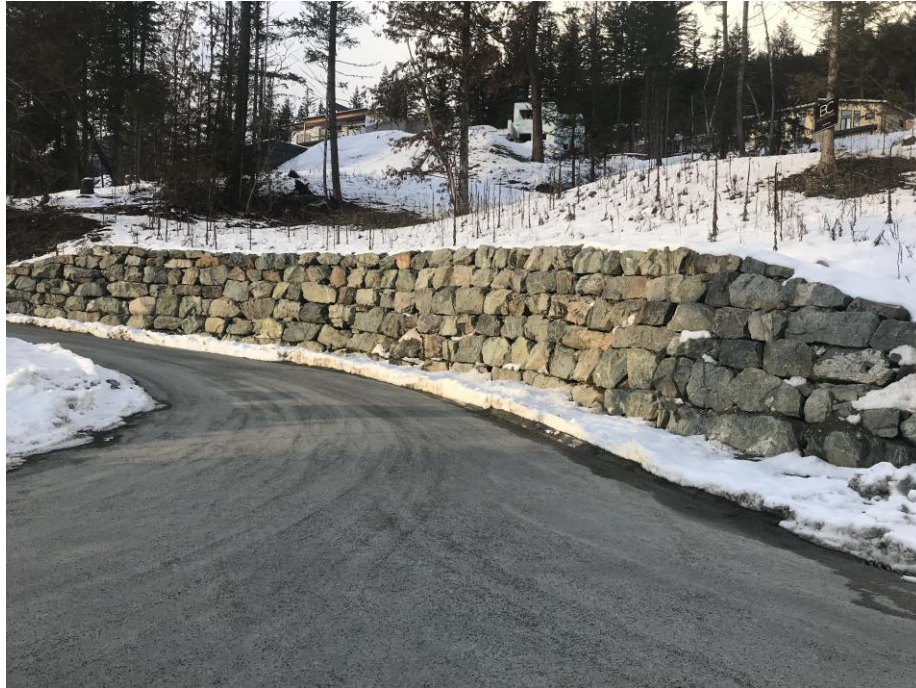
Figure 1: Lower Road Rock Wall
