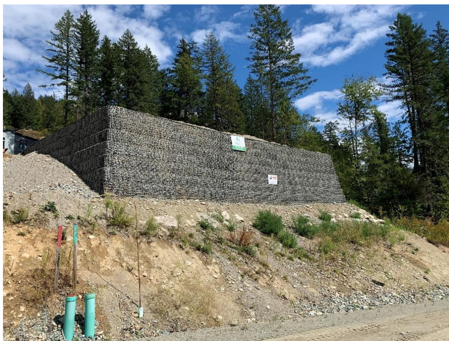
Figure 1: Photo of retaining wall located at 7665 Cerulean Drive taken on October 9, 2020
