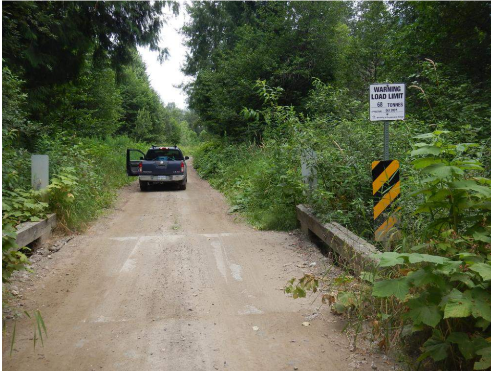
2km road runs beside the Ryan River and small bridges cross several creeks
