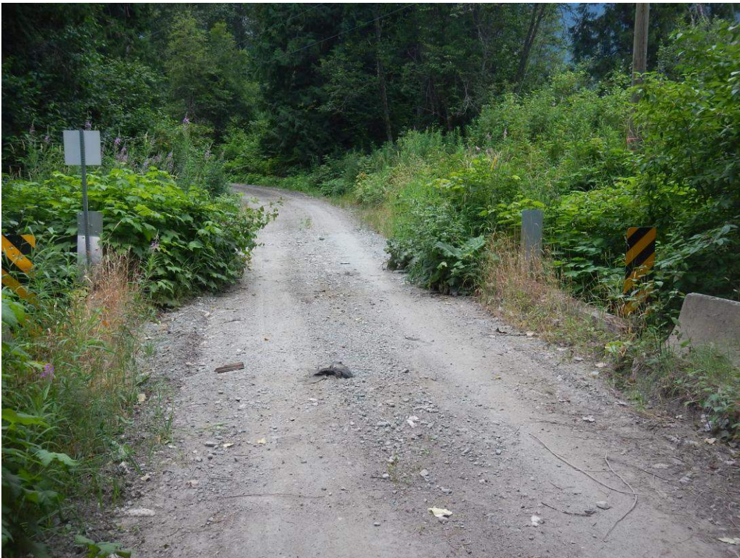
2.8 km a 3 metre long bridge. At 3.0 km the road begins to climb steeply
