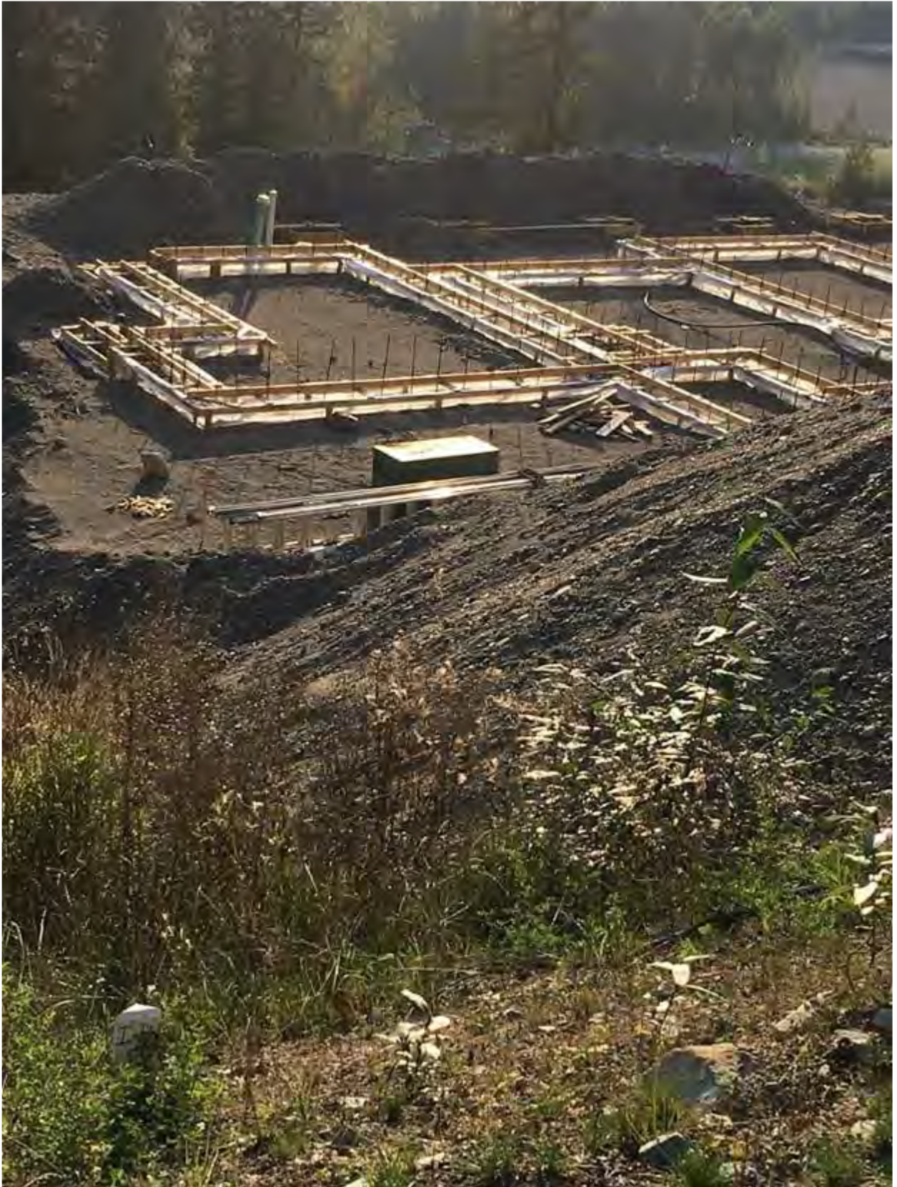
Photo B: # 7665 taken from corner of # 7663 at street level (Cerulean Drive)
