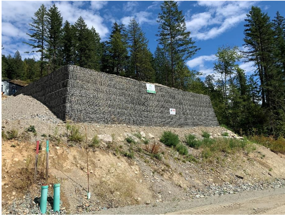
Figure 1: Photo of retaining wall located at 7665 Cerulean Drive taken on October 9, 2020
