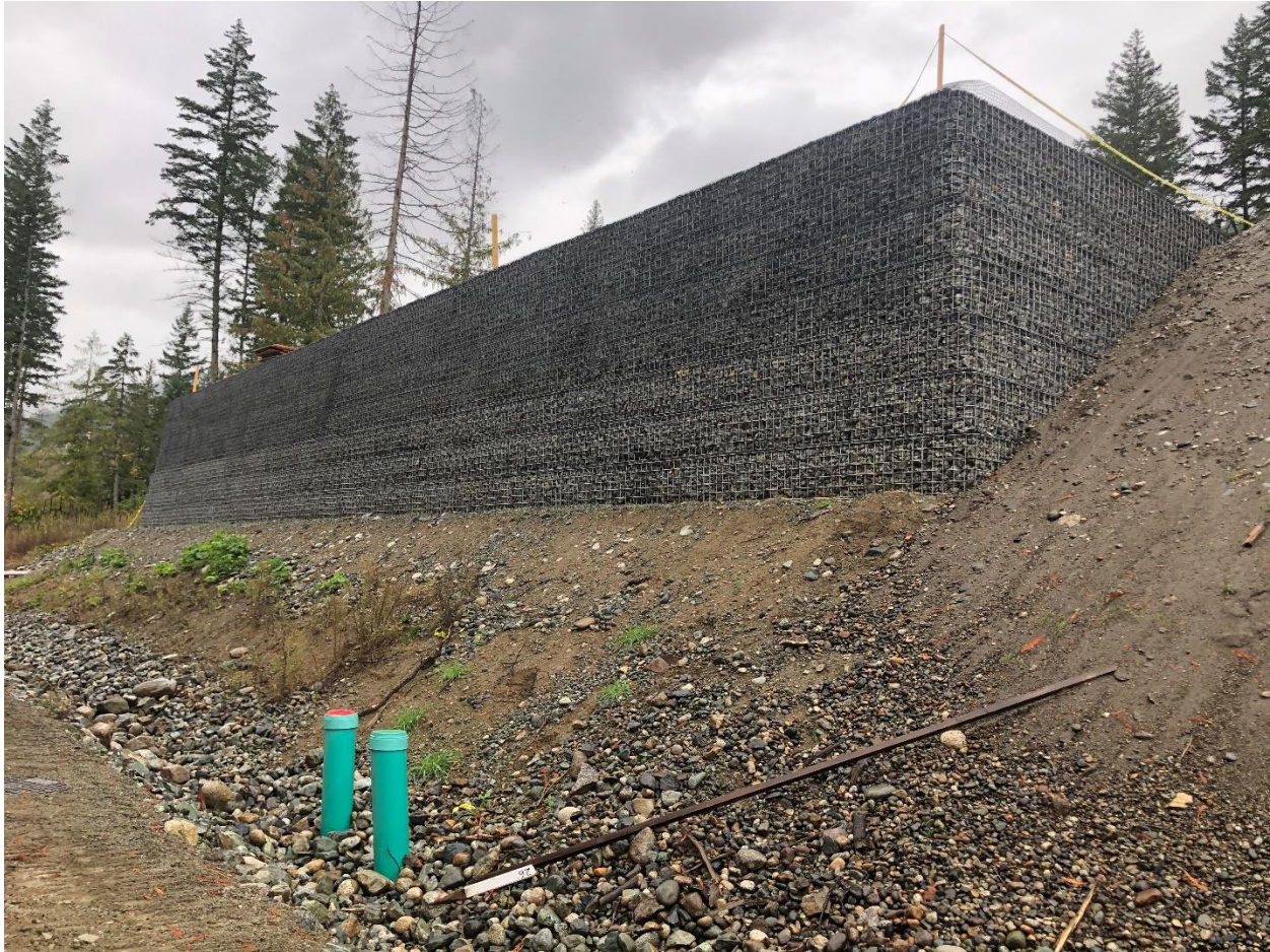
Figure 1: Photo of the retaining wall on the subject lands.
