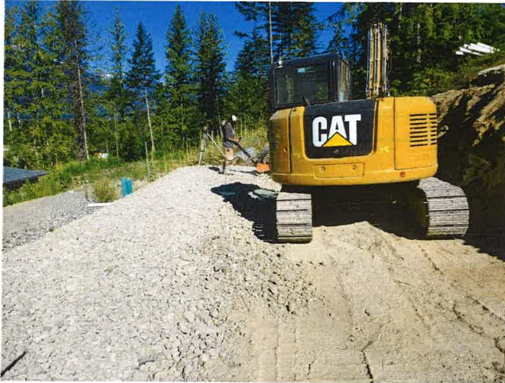
Photograph 1 – Subgrade Preparation
