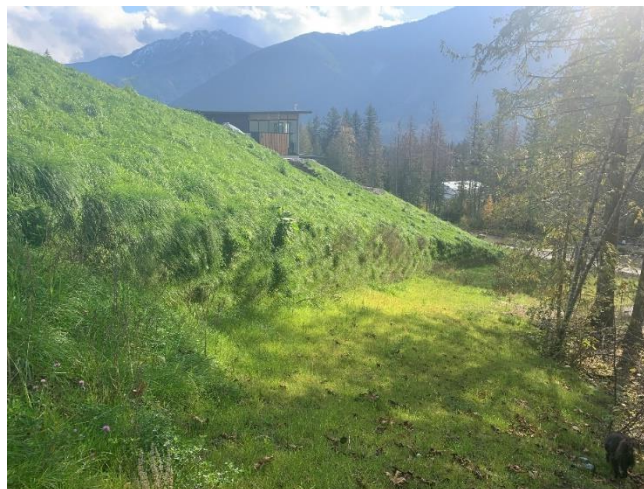
Figure 4: Photo of existing Sierra Earth Mechanized Wall located on the west end of the subject lands submitted by the Applicant.
