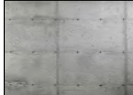
NATURAL ARCHITECTURAL FINISH CONCRETE ENTRY FOUNDATION WALLS
