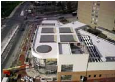
(Fig. 2.3) A combination of two public roads and two private fire lanes provides full perimeter access to this building.
