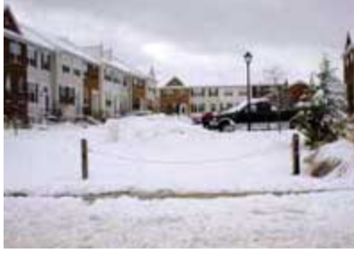
(Fig. 2.7) The same paver block access lane as shown in figure 2.6, but covered with snow. Access is blocked by a mound of snow plowed from the adjacent parking lot.
