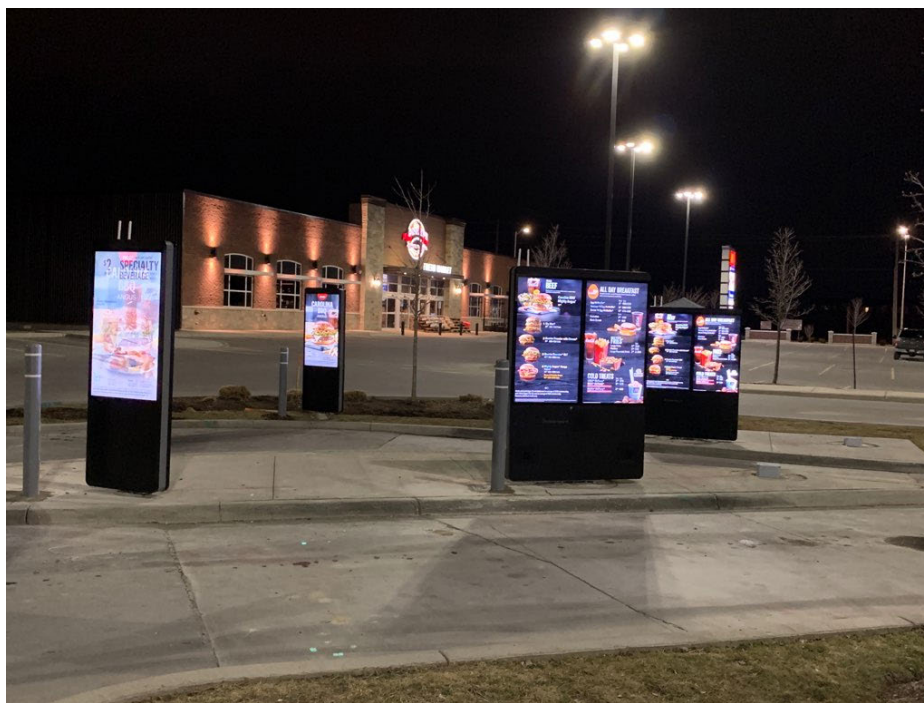
Example of a completed dual lane site from a recent installation.
