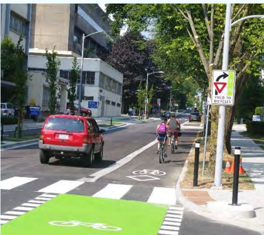
Figure 7: Example of a Cross-ride Pavement Marking with Conflict Paint and Cycling Stencils (Vancouver, BC)
