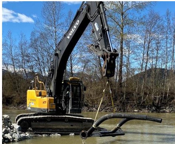
Figure 5 – Reinstalling Diffuser assembly
