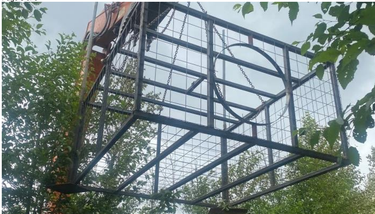
Figure 7 – Beaver box culvert protection
