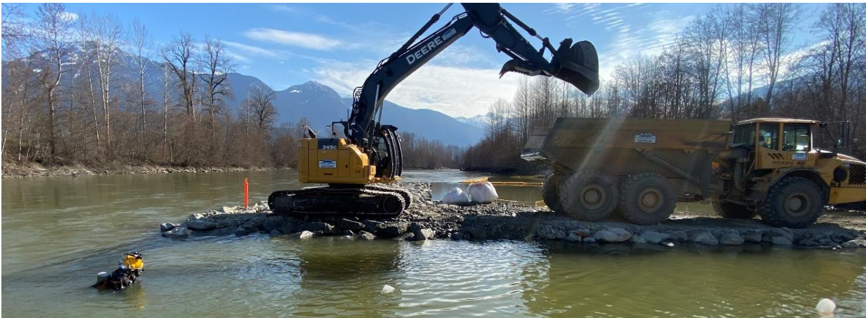
Figure 3 – Diver locating outfall diffuser ports and aiding excavator
