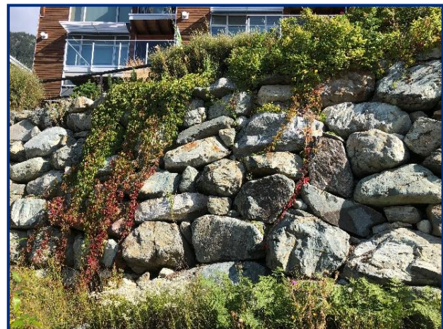
Retaining wall is made with natural building materials and visual impact is minimized with natural landscaping.
