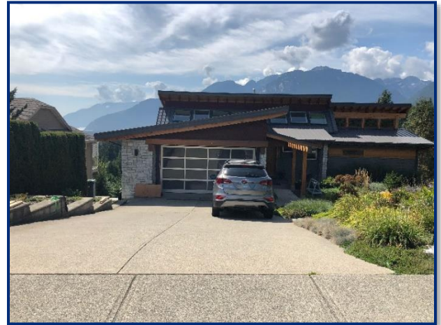
Sloped driveway reduces grading.
