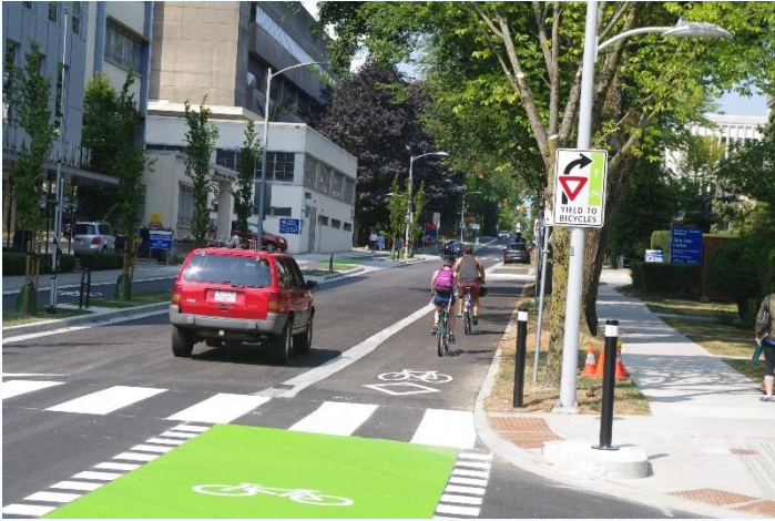
Figure 5: Example of a Cross-ride Pavement Marking with Conflict Paint and Cycling Stencils (Vancouver, BC)
