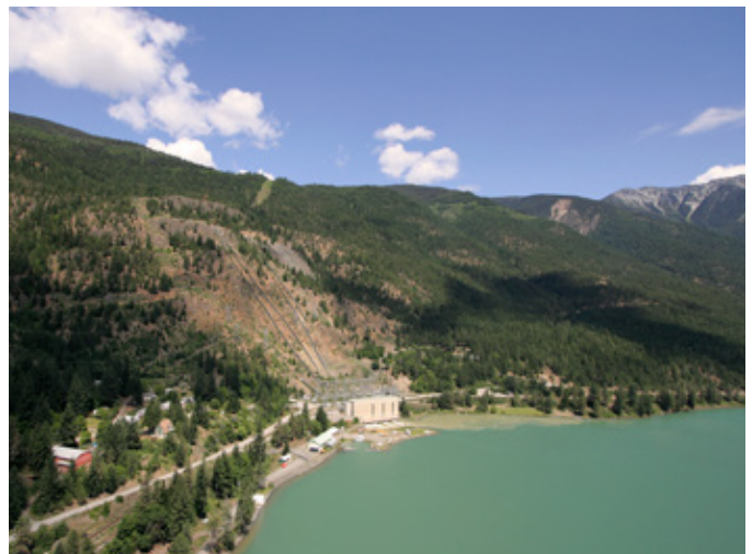
Bridge 1 power house, located approximately 300 kilometres north of Vancouver.
