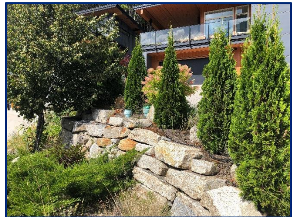
Small well-landscaped retaining walls used to maintain the natural topography and reduce grading.
