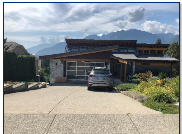
Sloped driveway reduces grading.
