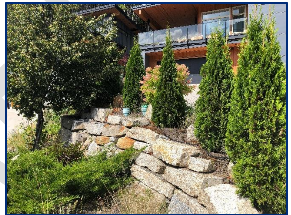
Small well-landscaped retaining walls used to maintain the natural topography and reduce grading.
