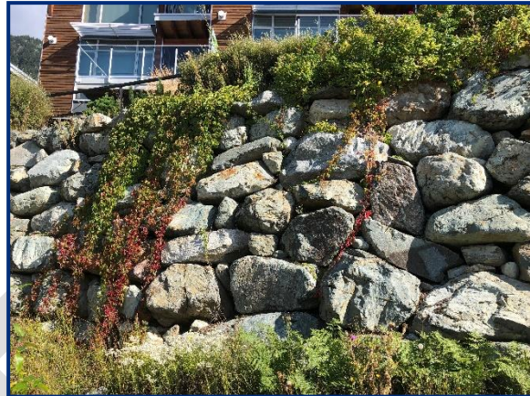
Retaining wall is made with natural building materials and visual impact minimized with natural landscaping.
