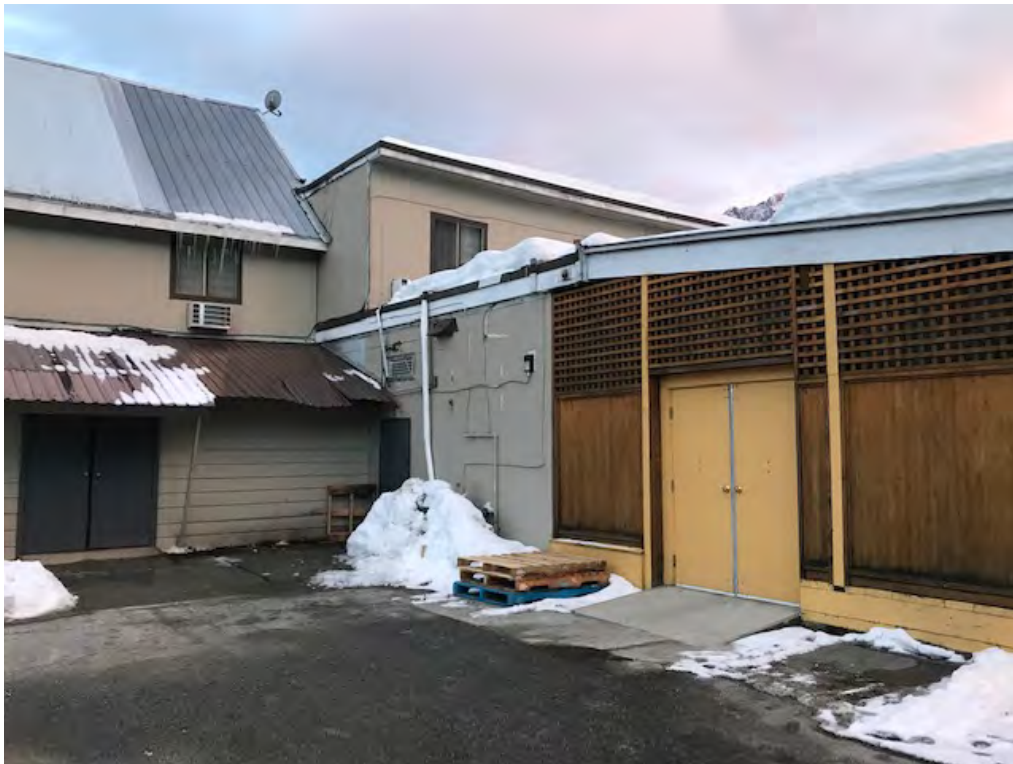
Rear – Covered Storage
