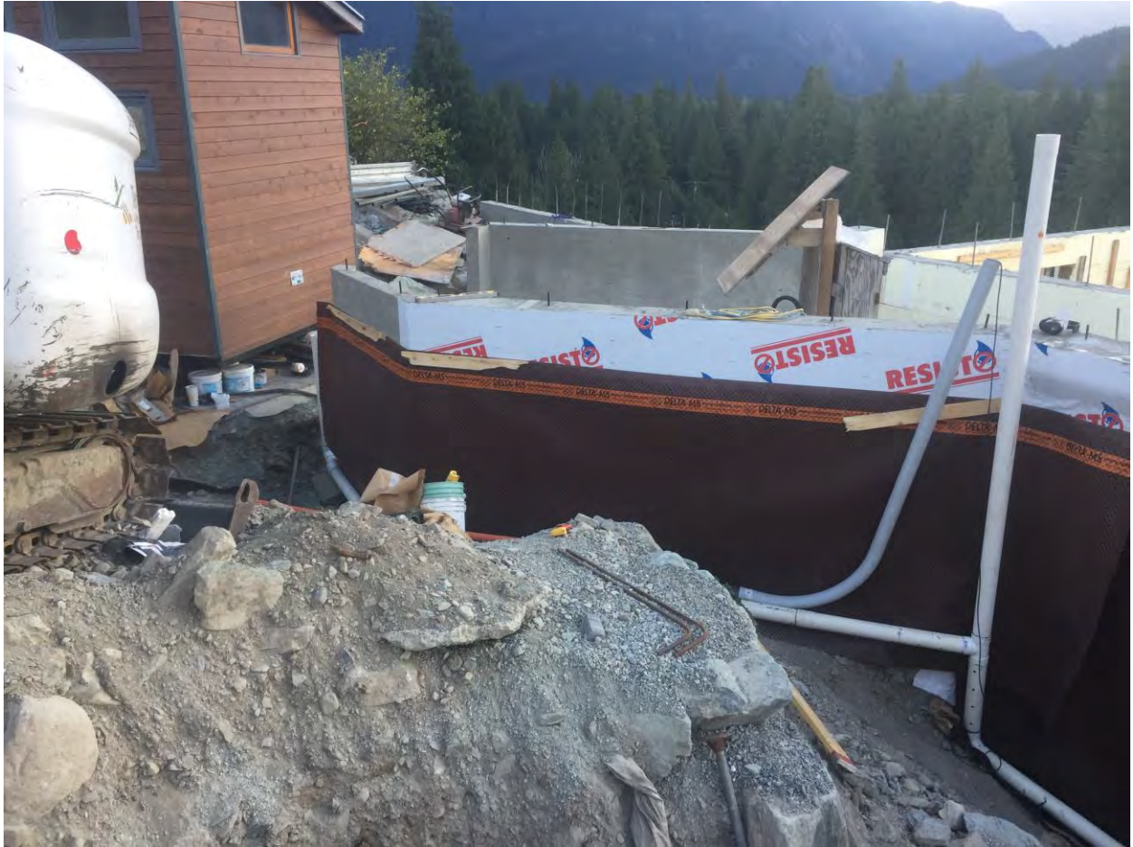
Foundation Looking East with Site Office on left
