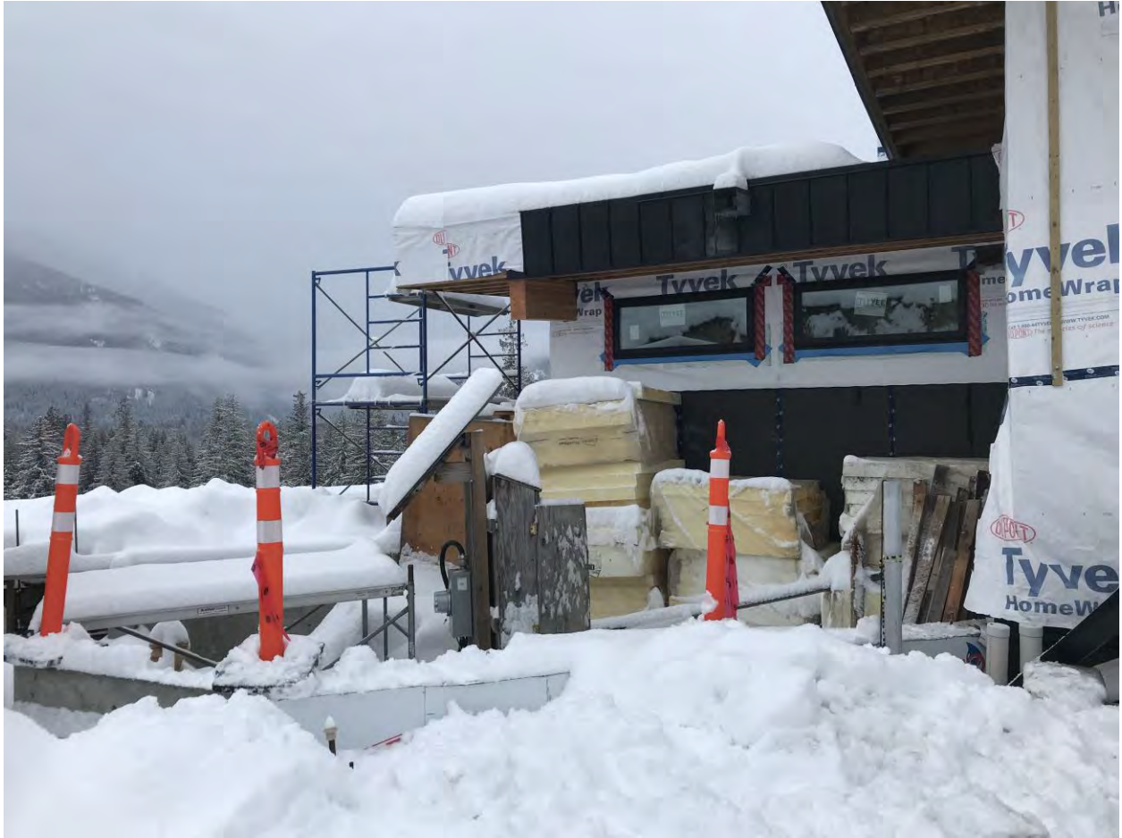
Front Elevation looking Northwest - foundation of garage marked with orange cones
