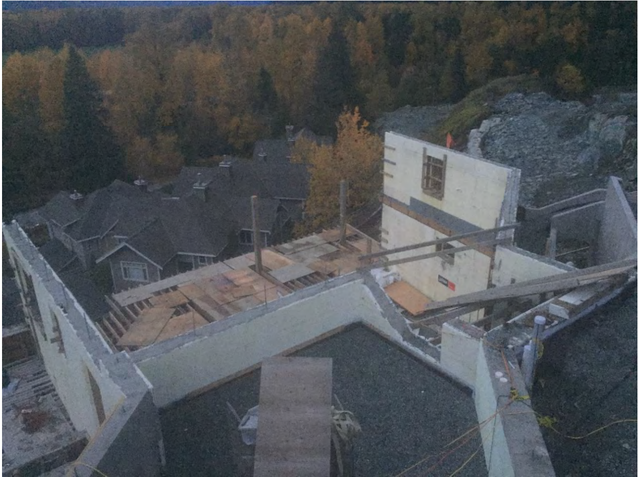
Front Elevation looking Northeast with garage foundation outline in foreground
