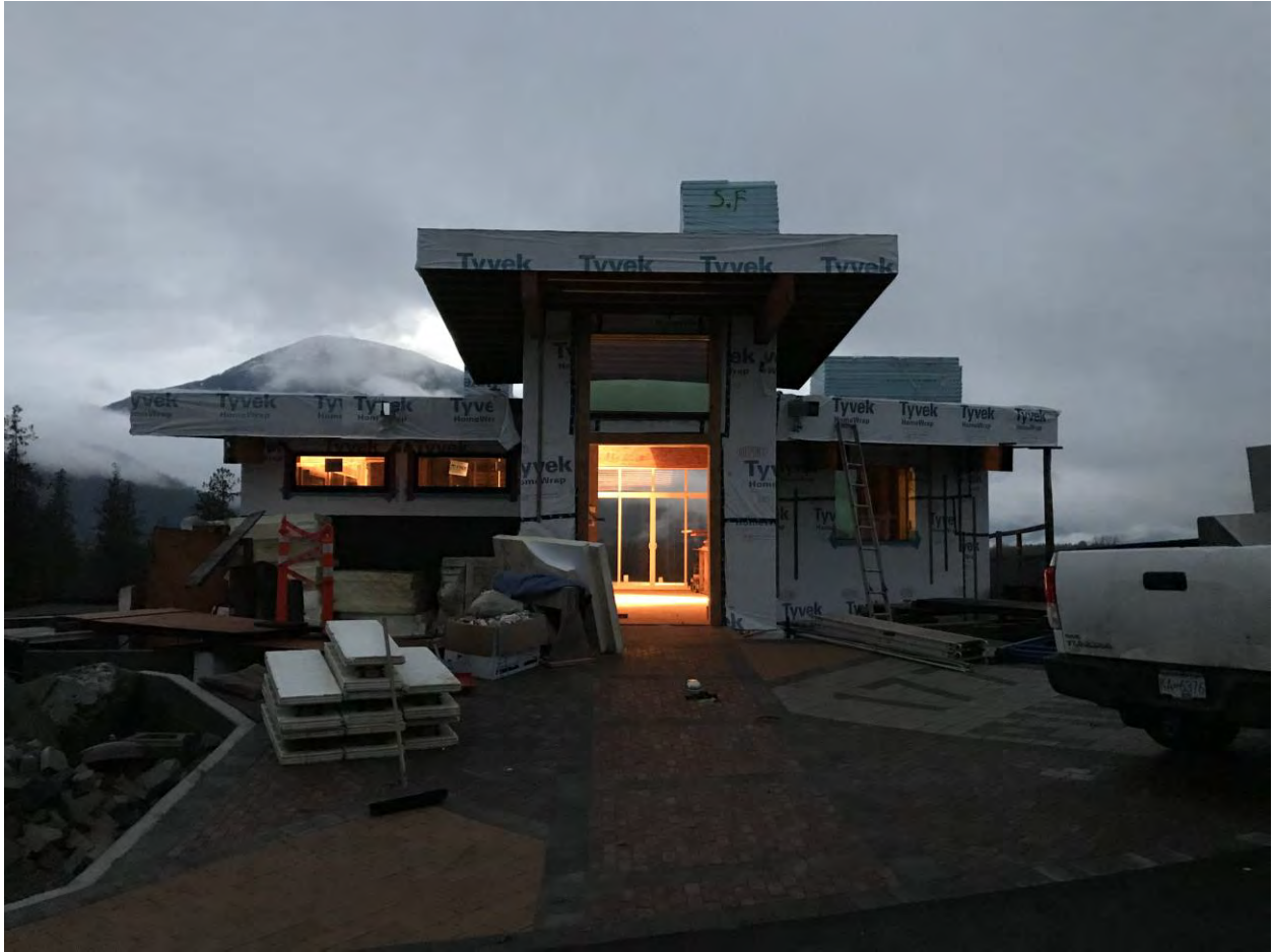
Looking North at the front elevation
