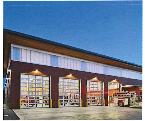
SILGA -- Southern Interior Local Government Association: Town of Osoyoos for the Osoyoos Fire Hall Courtesy: Wood Design Awards in BC
