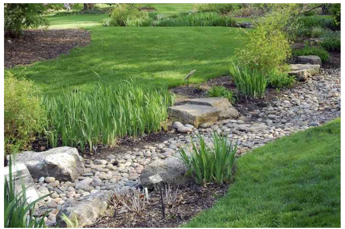
3 BIO-SWALE Stormwater is purified through air exposure and plants bio-filtration.
