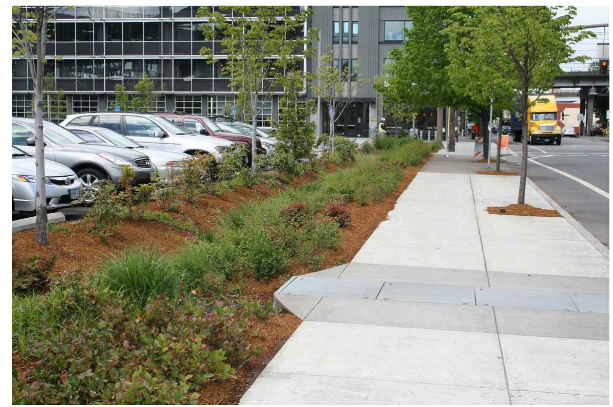
2 BIO-FILTRATION BEDS Filtration beds play a key role in reducing the amount of runoff and increasing water quality.
