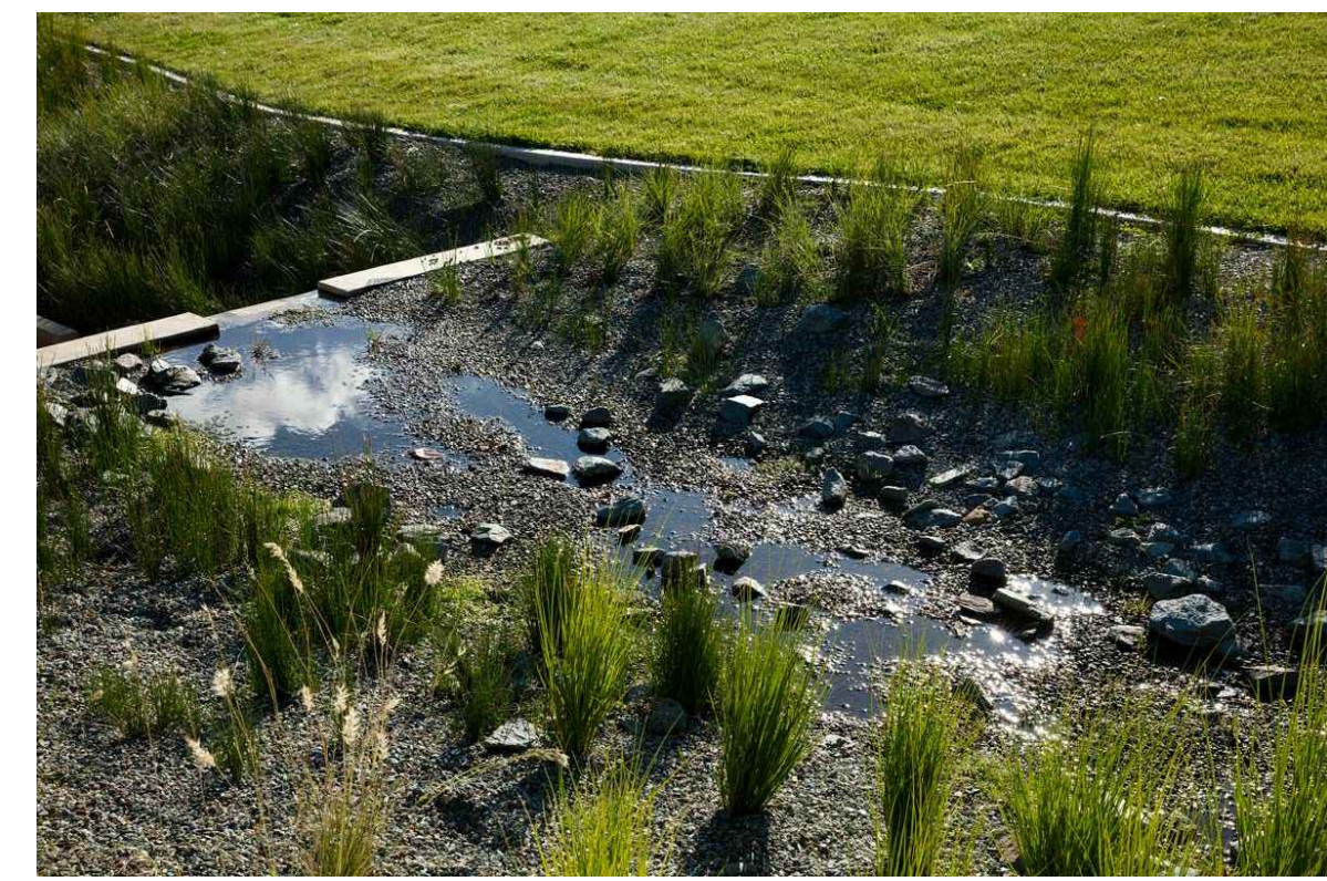
1 STORMWATER DETENTION POND Strategic ponds are located throughout the project to allow natural water infiltration in storm events.
