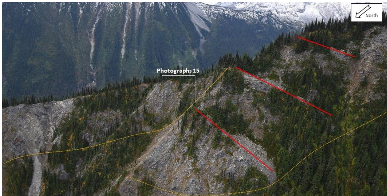
Photograph 17 Right: northeast side of Source ID 2a, showing lineaments (red lines) and associated slope deformation parallel to foliation, and inferred basal sliding surface (orange dashed line). Left: southwest side of Source ID 2b and inferred basal sliding surface (orange dashed line).
