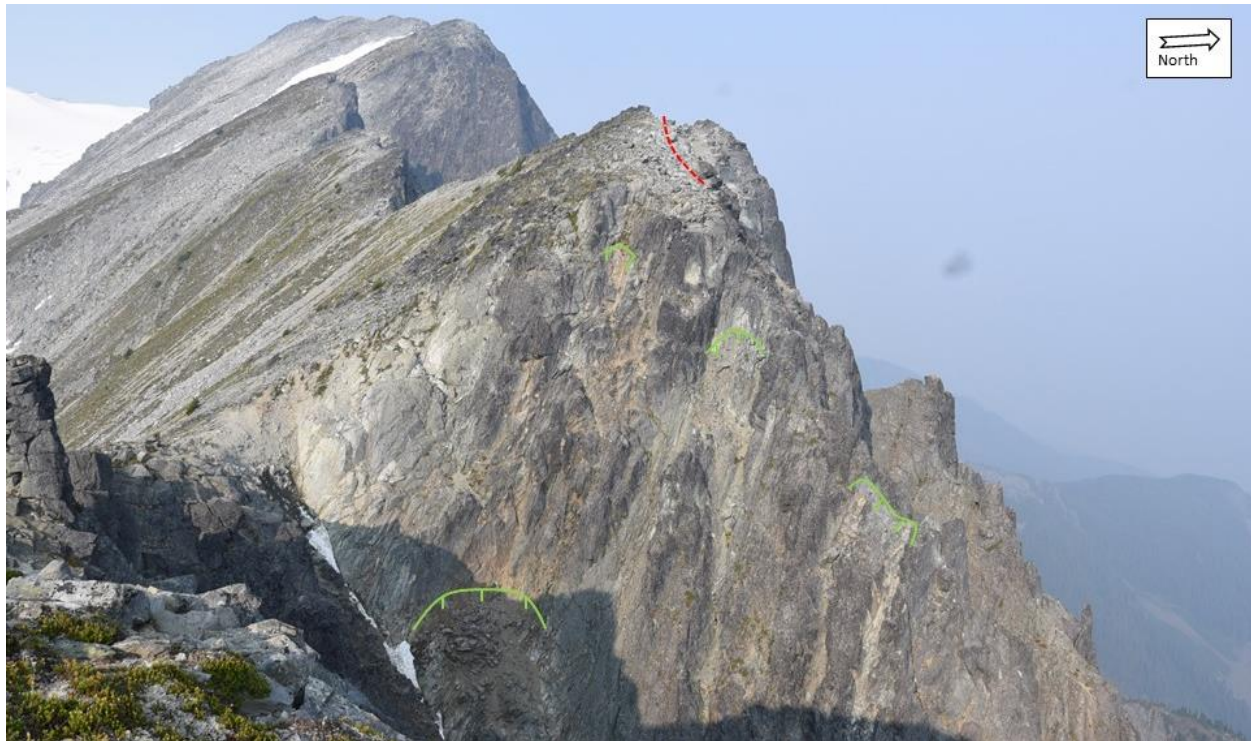
Photograph 31 Minor rock fall scars (green lines); and tension crack (red dashed line) defining a potential instability (Source ID 12).
