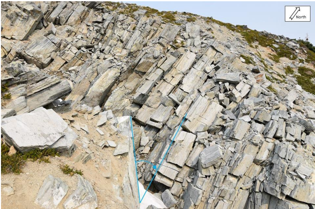
Photograph 6 Disturbed and dilated rock mass (Source ID 1a) with tilted blocks along foliation.
