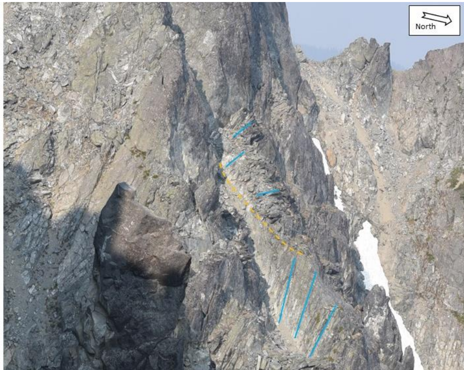
Photograph 37 Toppling mechanism generating a disturbed mass whose interpreted basal sliding surface (orange dashed line) corresponds to the location where undisturbed foliation planes (blue lines) become tilted.
