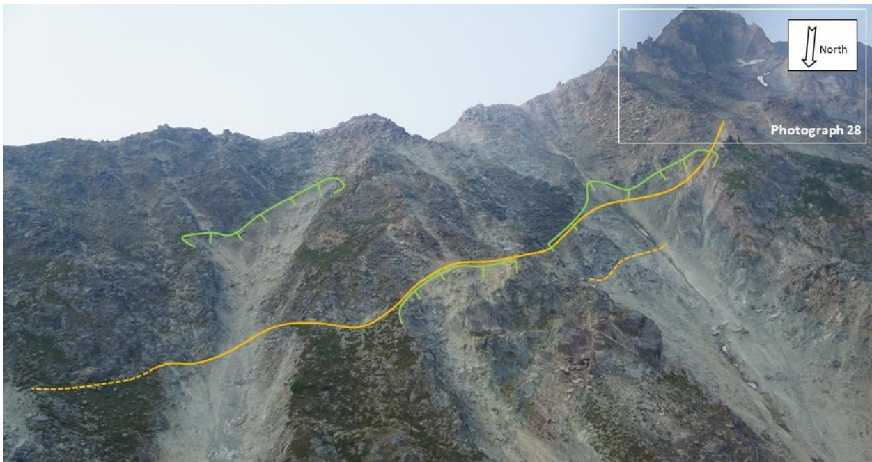
Photograph 7 Scars (green lines) of small landslides initiating on the edge of the disturbed mass (Source ID 1a) and interpreted basal sliding surfaces (orange dashed line) of the disturbed mass.
