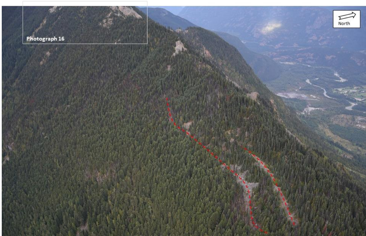
Photograph 12 Tension cracks (red dashed lines) subparallel to the ridge at Source ID 2c.
