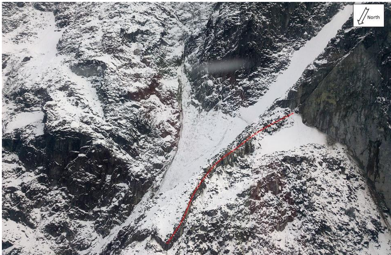
Photograph 34 Upper counter-slope scarp (red dashed line) of the July and September 2016 rock slide events.
