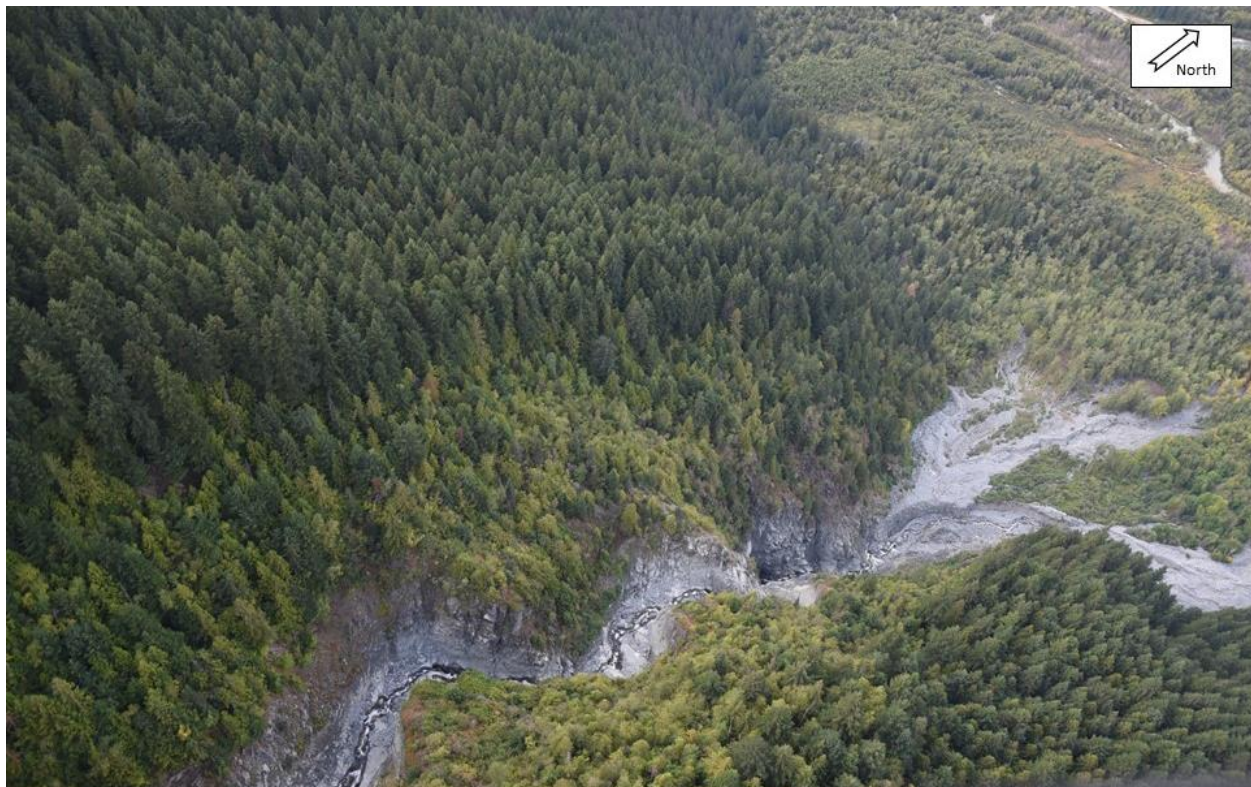
Photograph 44 Deeply incised gully on the lower part of the debris flow path of Watershed B.
