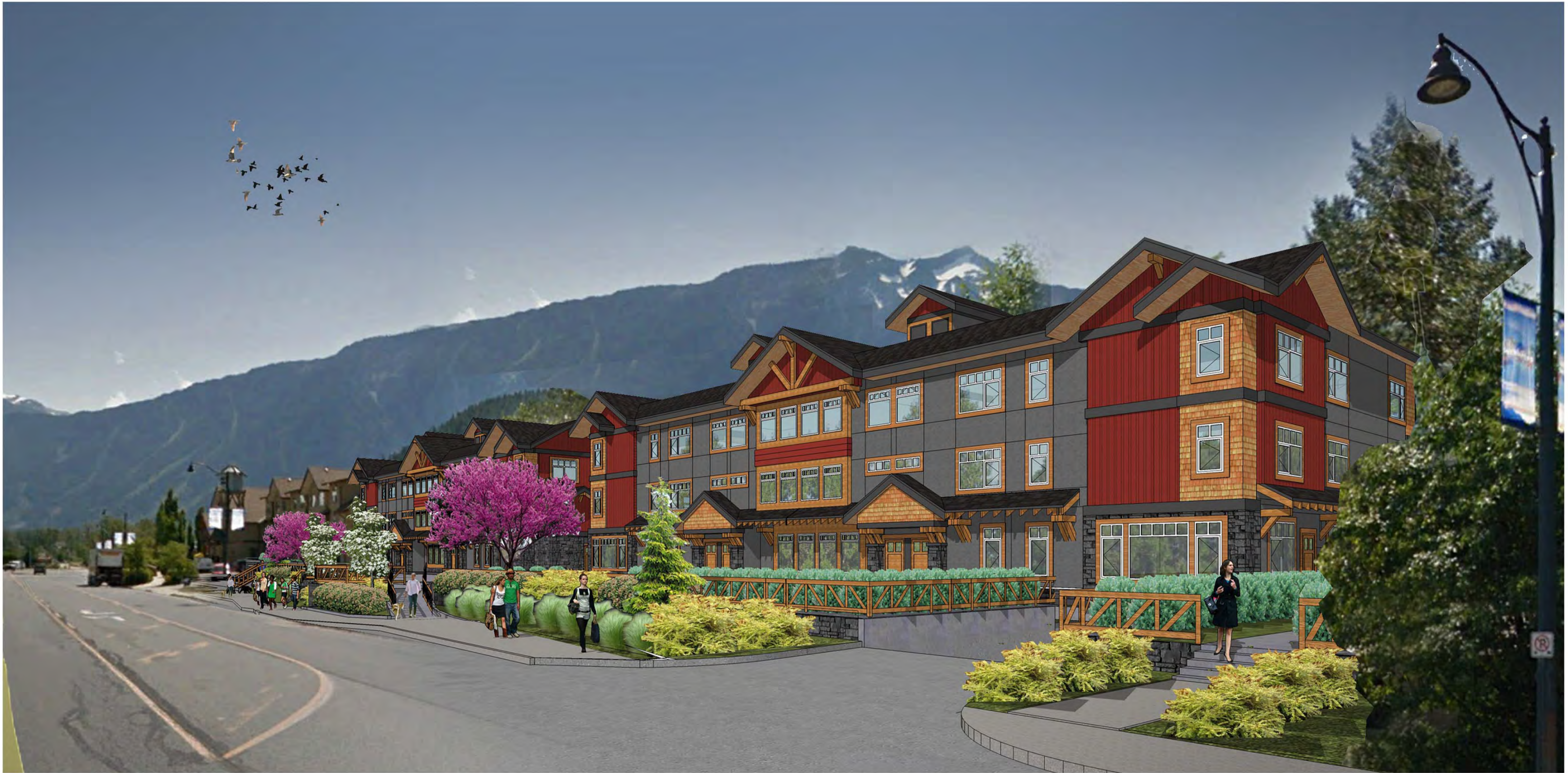
VIEW OF NORTH WEST ELEVATION
