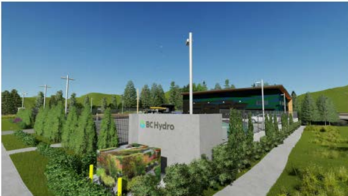
Figure B – View from Aster Street (southwest)
