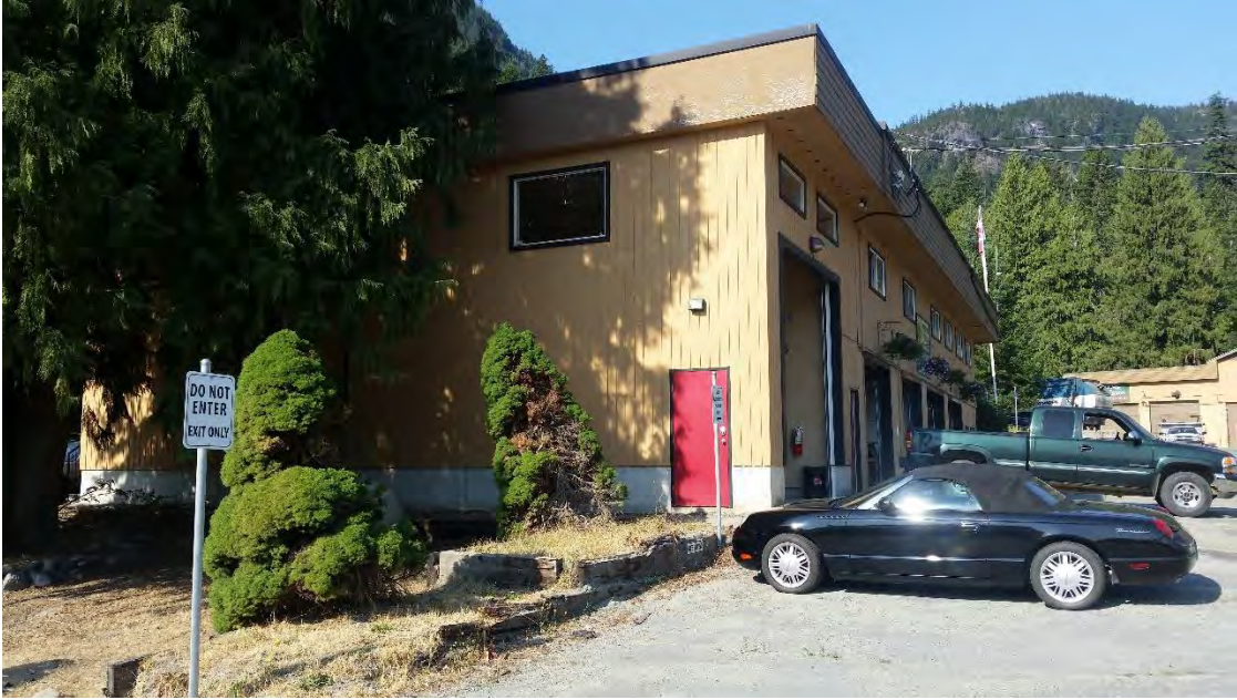
Building Side View
