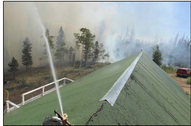
Figure 20. Both photos are from the Beaver Creek Fire in Colorado. Photo credits: Wardner’s Type III Incident Management Team. Left: the success was attributed to the combination of efforts of the homeowner with construction and mitigation work and the firefighters with water tanks, pumps, hose, and sprinklers. Right: exterior sprinklers on a home raise the relative humidity around the structure.
