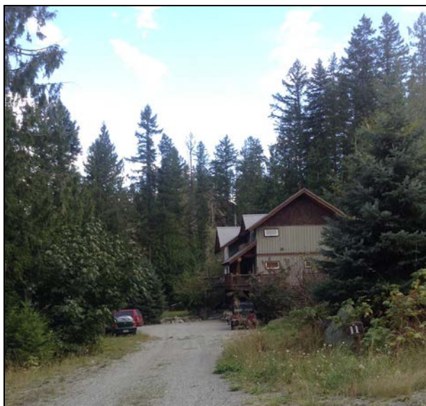
Figure 17. Property and homes are in a range of FireSmart compliance. Left: typical house in more rural parts of the study area. Right: typical house within the Village boundary and more developed portions of the study area. Note the metal roof, which is FireSmart compliant, but there is not sufficient defensible space.
