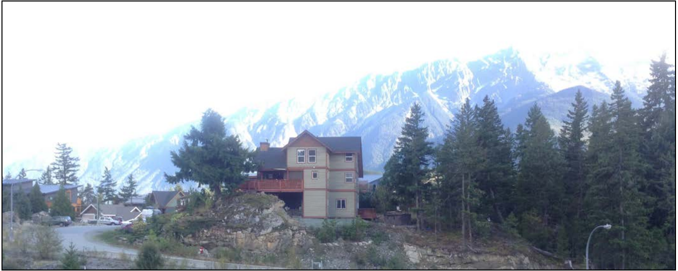
Figure 18. Typical home in the Benchlands. Roofing is FireSmart compliant, though open decks provide locations for embers to get trapped and ignite the home.
