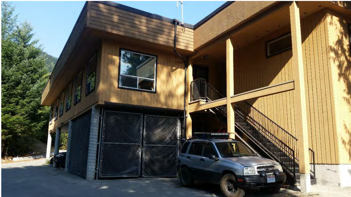
Building Rear Side View (proposed addition location)
