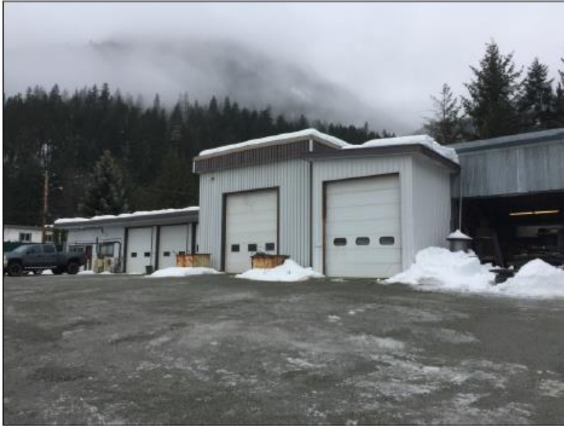
Photograph 1: Site building – looking southwest
