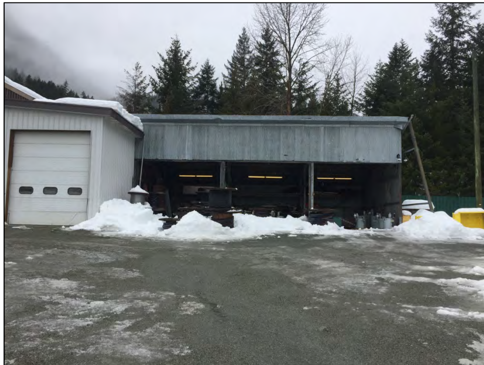
Photograph 2: Storage shed on west portion of the Site – looking west
