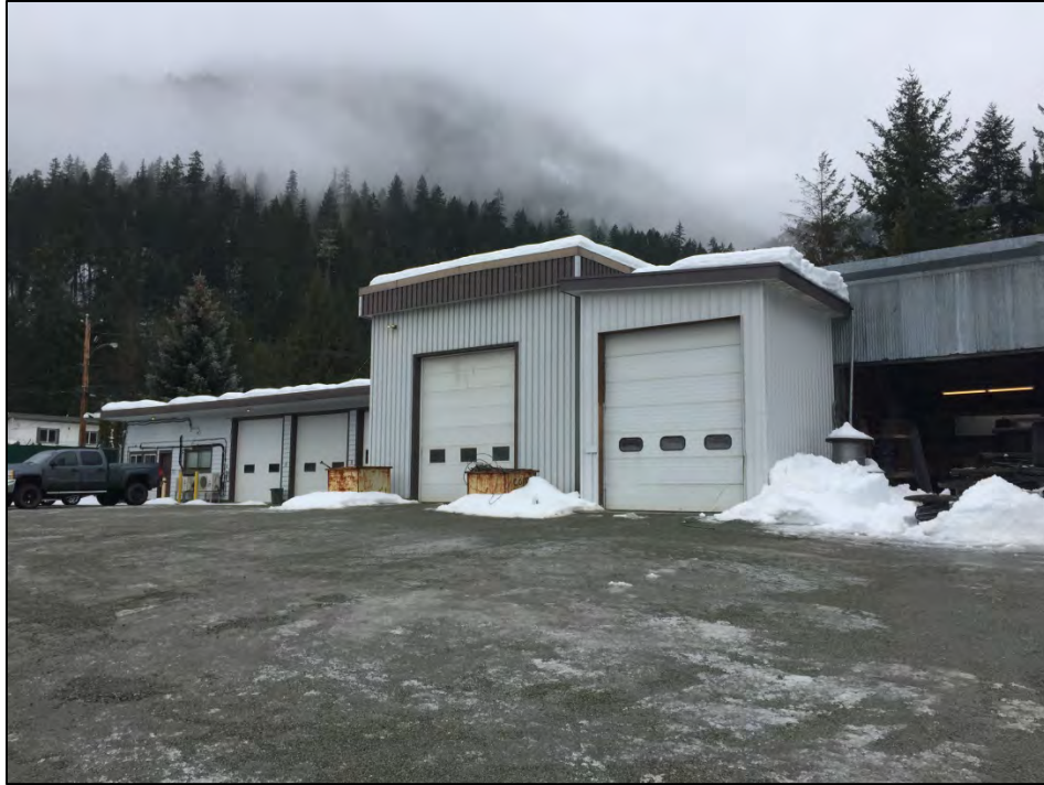
Photograph 1: Site building – looking southwest
